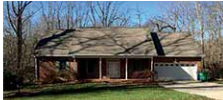
102 OAKLAWN RD - Need room for a growing family! This is it! Home features 4 bed 3 full baths, beautiful hardwood floors, LR, dining room, big open kitchen, pantry, and 2 car garage. Finished basement with huge den/game room. Tons of closets! Home sits on over 2 acres and has a deck and storage building. Make your appointment now! $249,900
