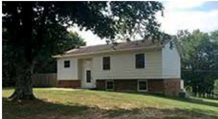
802746- 357 HERRING ST - Nice 4 bedroom home with 2 full baths, above ground pool, very nice two tier deck, 22x14 det. garage/workshop out back with electricity, fresh paint inside and out! Move in ready! 4th bedroom and 2nd bath in basement. Very well maintained, all kitchen appliances remain! Home located near end of street in culdesac. Make your appointment today! $123,500
