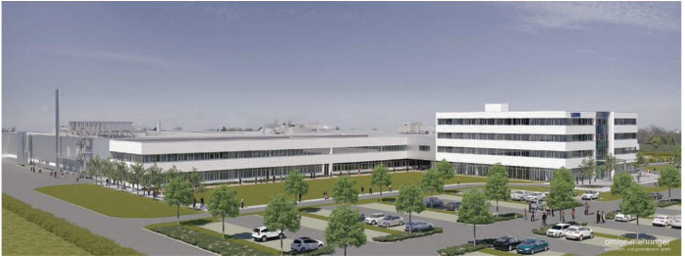
○ Leoni's 'Factory of the Future' will be erected on a 134,000m 2 -sized area (computer graphic)
