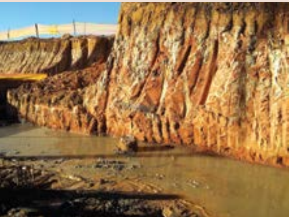
Various in-situ soil types posed a challenge for effective drainage.
