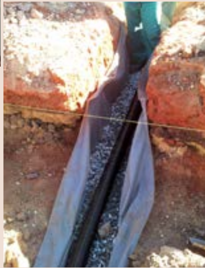
Geomesh used in a conventional drain system.
