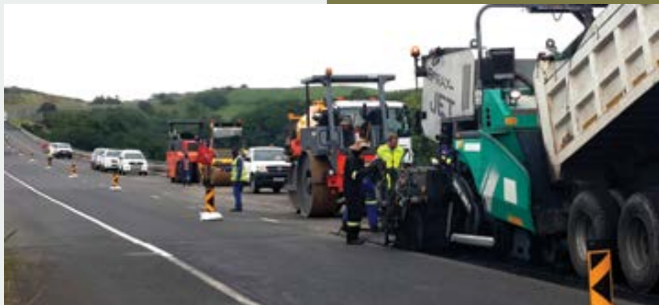
BOTTOM RIGHT: The tack coat being sprayed onto the milled surface.
