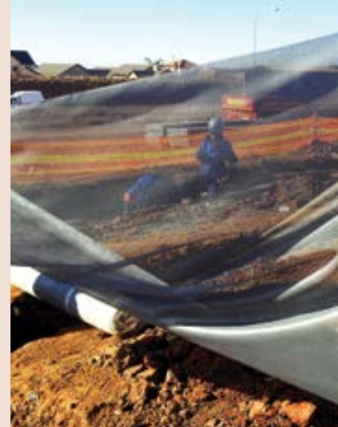
Geomesh has larger openings than woven tape to provide non-clogging drainage.
