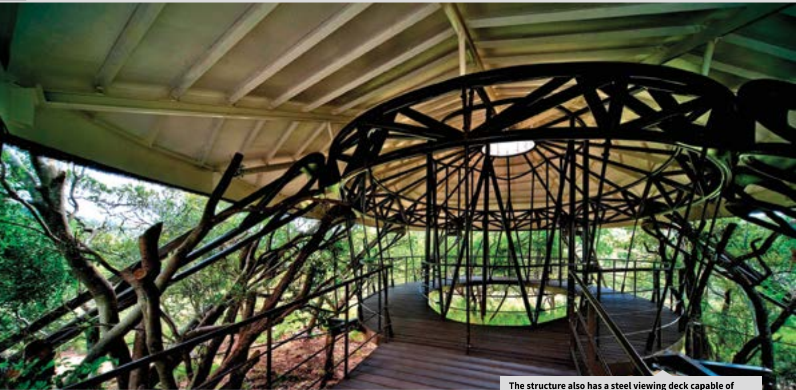
The structure also has a steel viewing deck capable of taking a maximum of 33 people. It is suspended from underneath the lattice girder and the roof using steel ties.
