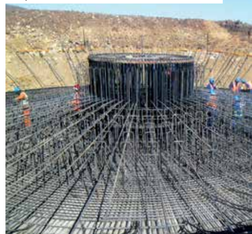
Steel reinforcement in progress on a base at Noupoort Wind Farm.
