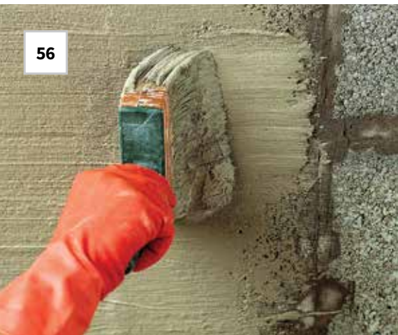
ABOVE: Planiseal 88 applied by brush to concrete surface.
