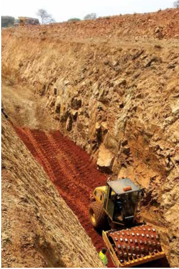
Clay core being processed at Katonga Dam.
