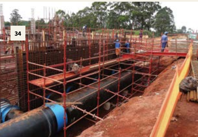
The Ashley Drive break pressure tank is under construction, when complete it will hold 20 mega litres of water.
