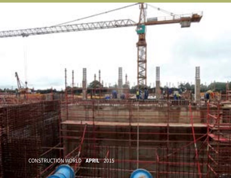
The Ashley Drive break pressure tank is under construction, when complete it will hold 20 mega litres of water.
