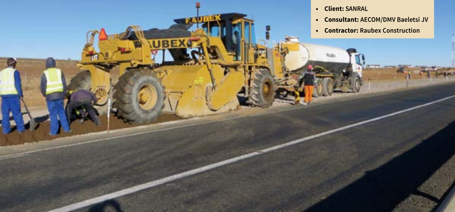
MAIN, LEFT: Base construction in progress & RIGHT: Sub-base stabilisation in progress.
