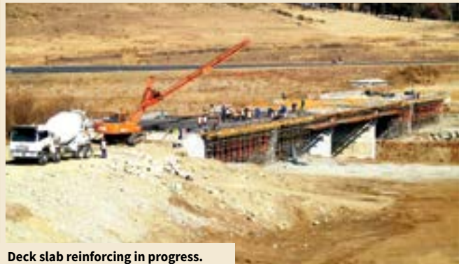
Deck slab reinforcing in progress.
