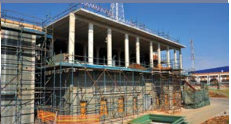
ABOVE: A workman finishes off one of the column/beam joints at MNT's data centre. BELOW: Phase II of MTN's Centurion data centre takes shape using Echo prestressed slabs.
