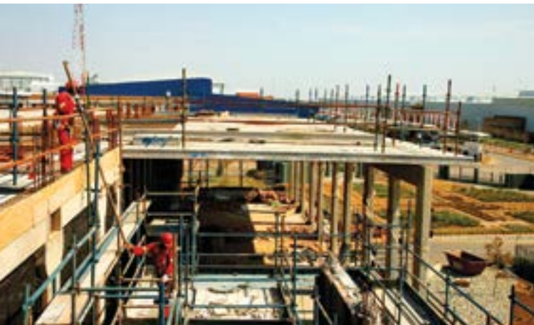
ABOVE: Echo's prestressed slabs are supported by concrete columns and precast beams. BELOW: Some of the installed Echo prestressed slabs of Phase II of the MTN data centre switch roof project.
