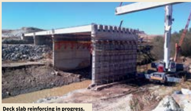
Deck slab reinforcing in progress.
