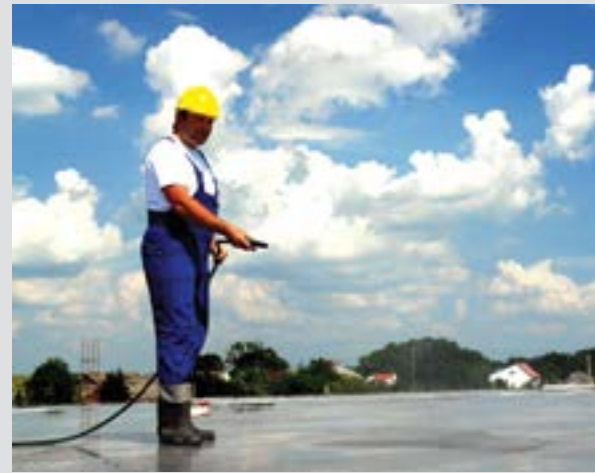
Incorrect curing methods still prevail in the South African construction industry, says The Concrete Institute.
