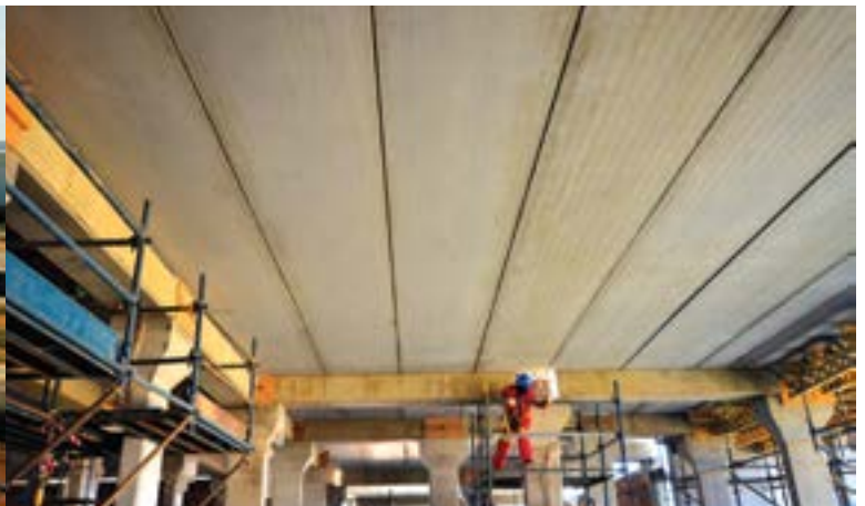
ABOVE: A workman finishes off one of the column/beam joints at MNT's data centre. BELOW: Phase II of MTN's Centurion data centre takes shape using Echo prestressed slabs.
