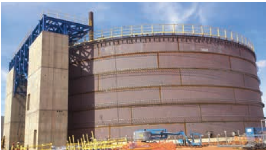
The Bokpoort CSP plant is suitable for base load generation because huge molten salt storage tanks are used to generate electricity for up to 9.3 hours during the night.
