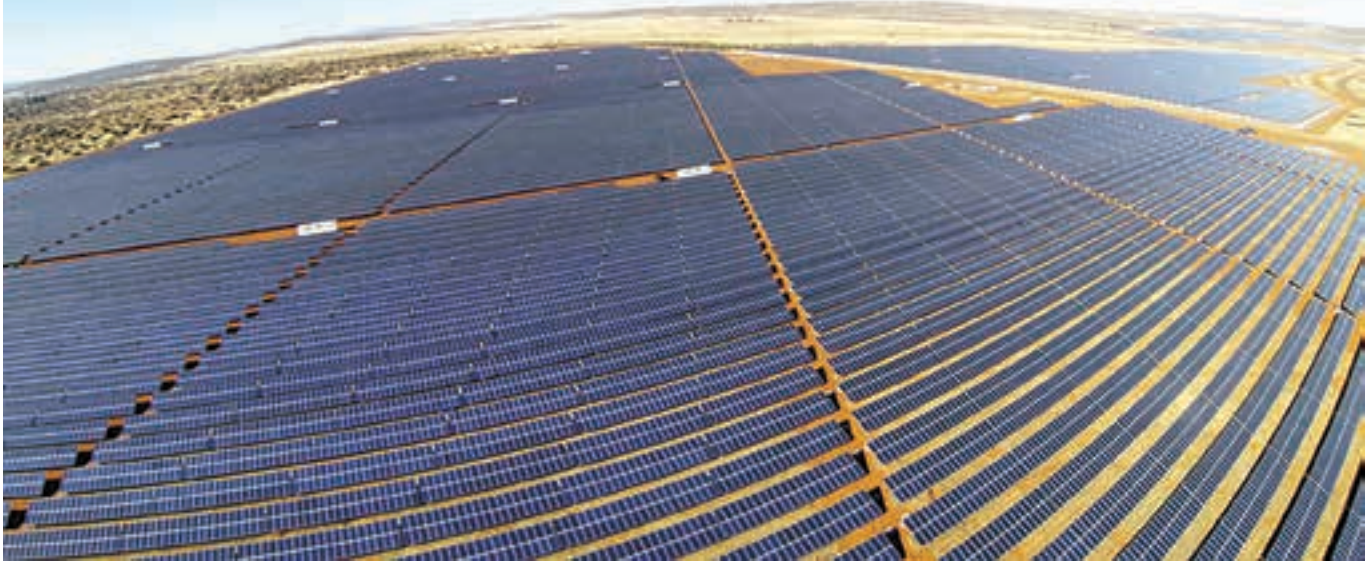
The 96 MW Jasper photovoltaic solar power project near Kimberley is the largest on the continent and can produce 180 000 MWh of energy per year. The CSIR has found that that renewable energy generation created net positive benefits of R0.8-billion during 2014.
