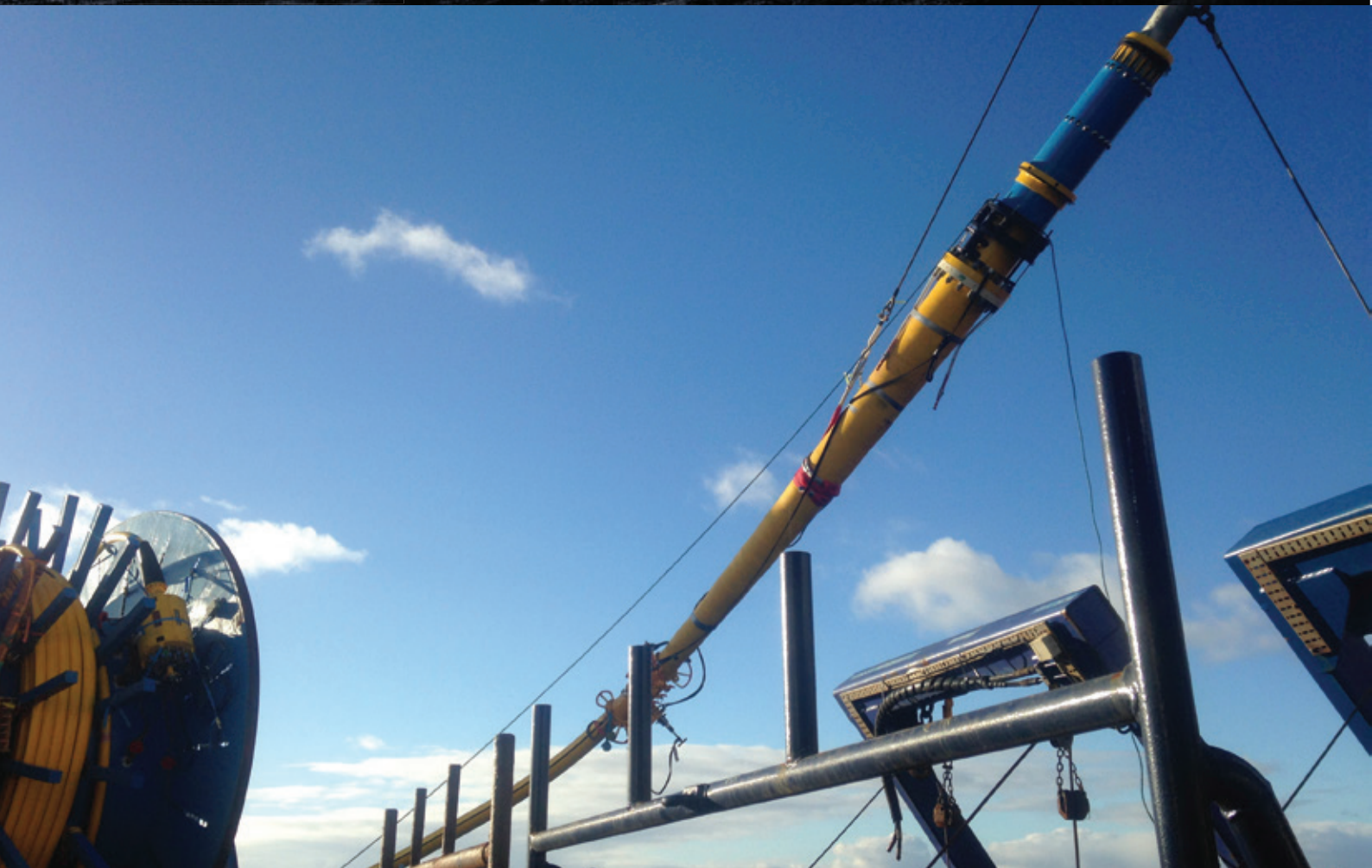
○ The connector being loaded onto the cable at Fukushima floating offshore wind farm demonstration
