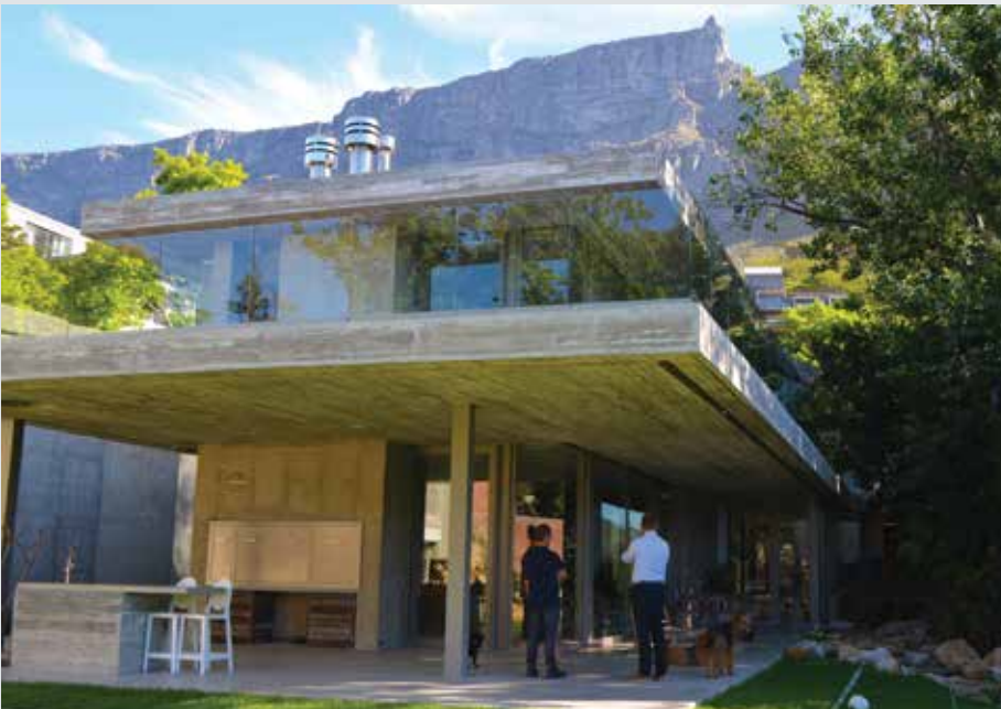
Glen Crescent House.
