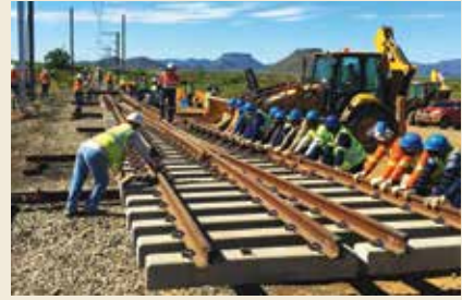
During training one of the female site engineers was promoted to construction manager.
