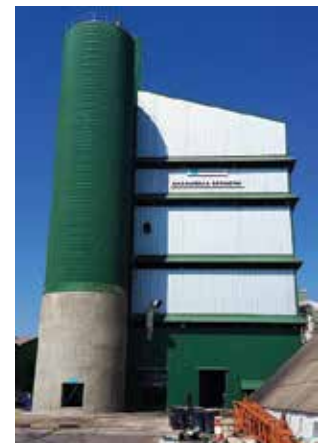
New refinery pan floor.
