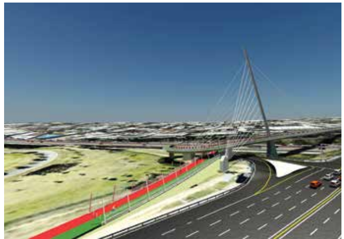
ABOVE: The Grayston pedestrian and cyclist bridge.
