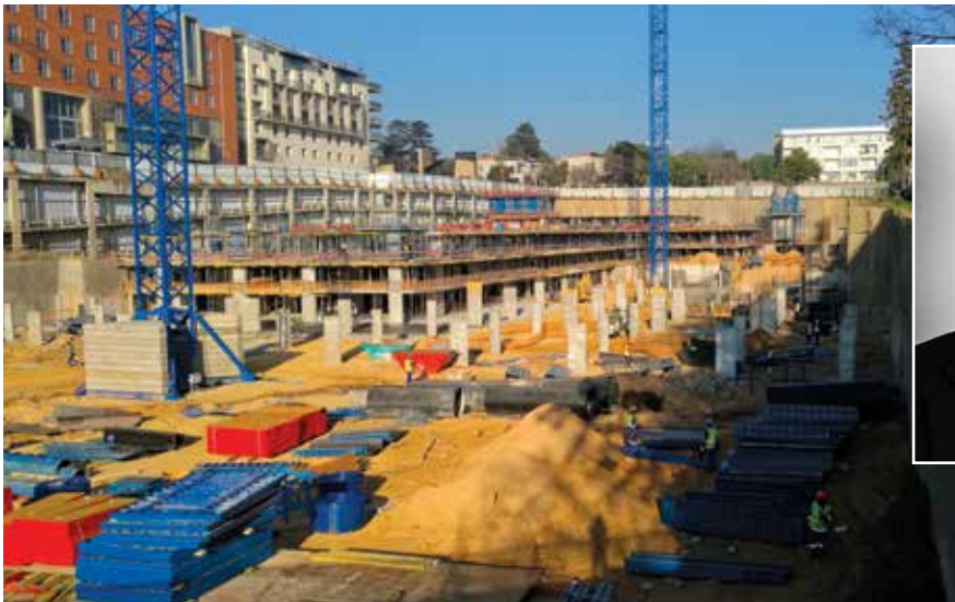
Current construction on One on Whiteley at Melrose Arch.
