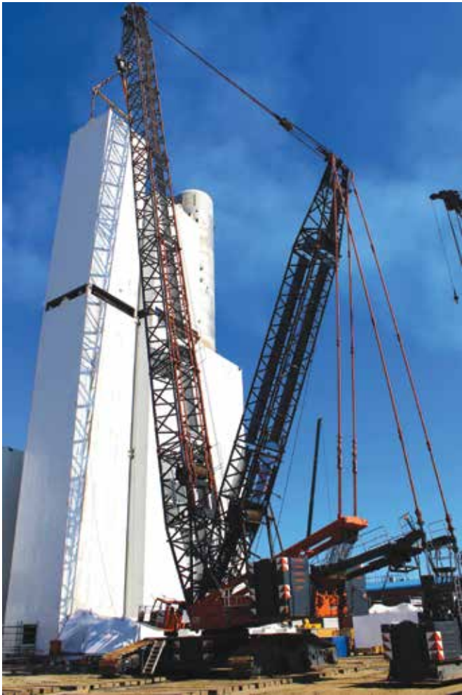
Most of the large components were lifted almost fully assembled.
