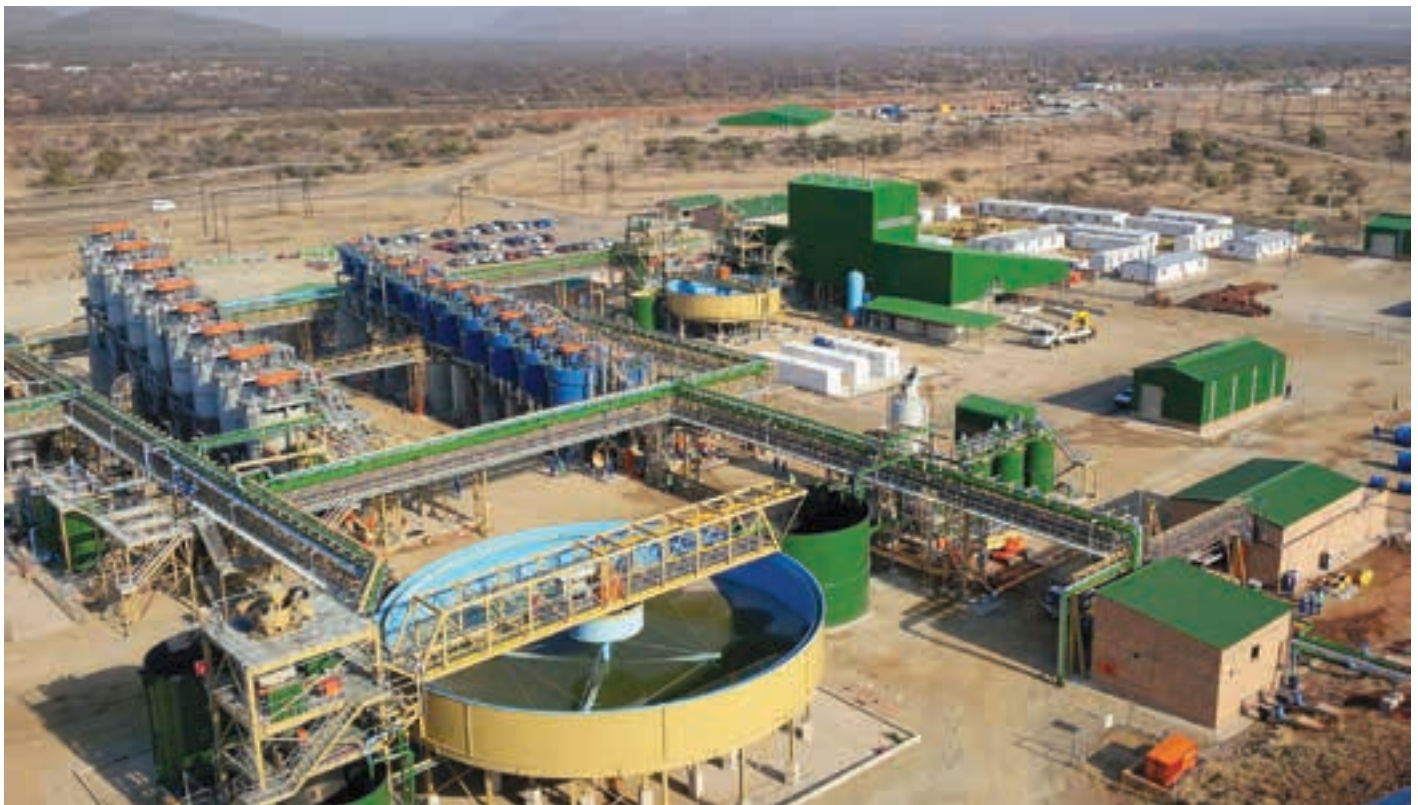
Maseve processing facility showing flotation circuit, concentrator and filter press (photo: Platinum Group Metals).
