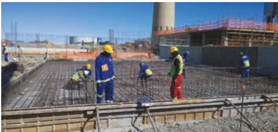
Preparing for a concrete pour at the furnace site.
