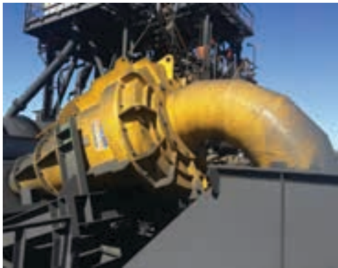
A Cavex® DMS cyclone installed in a coal application.
