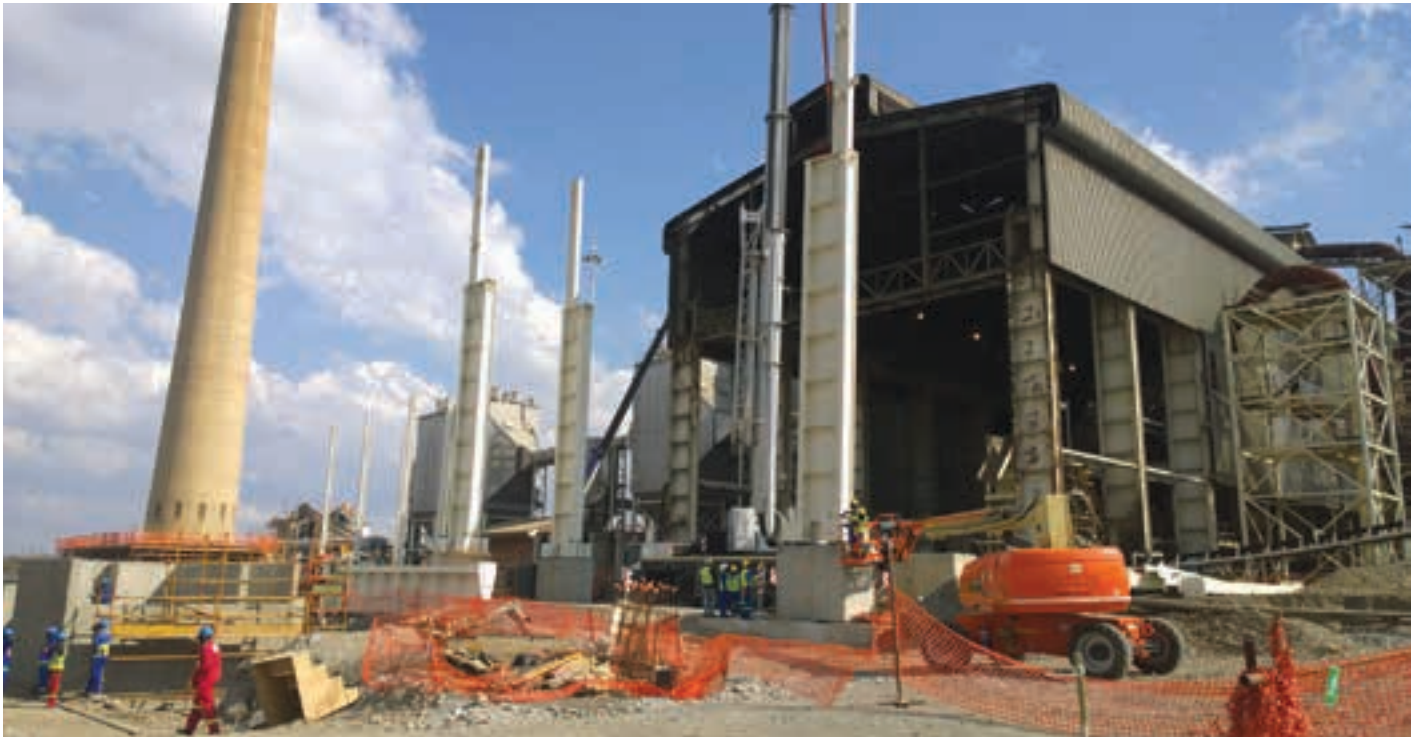
The new furnace at Northam Platinum's Zondereinde smelter operation under construction.
