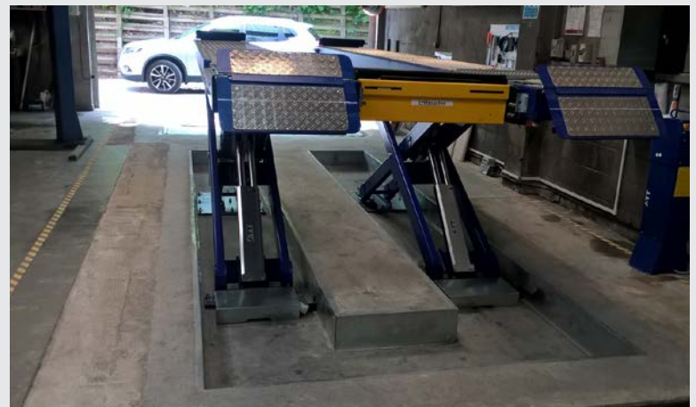
Jacking Beam Recess
