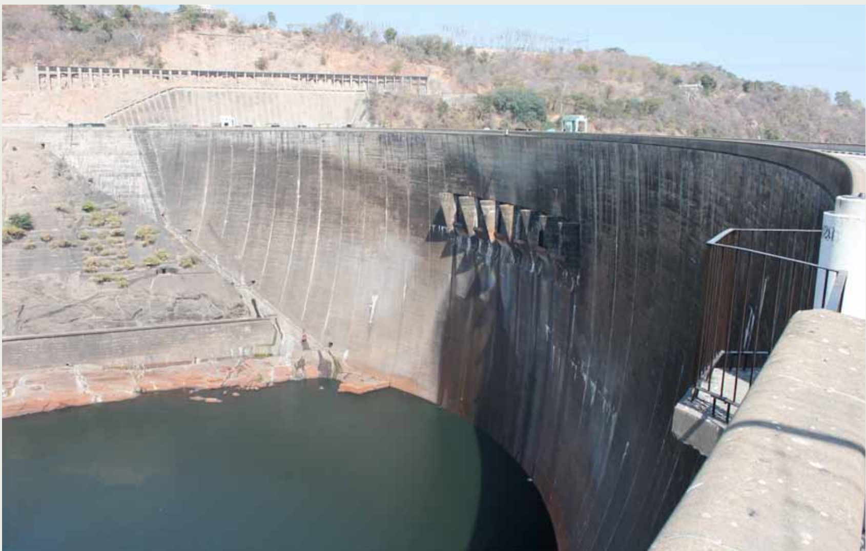
Kariba Dam in Siavonga, Southern Province
