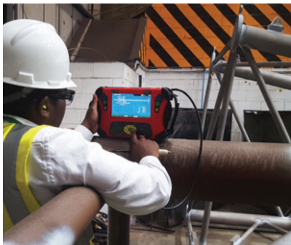
Pace crane structure inspection
