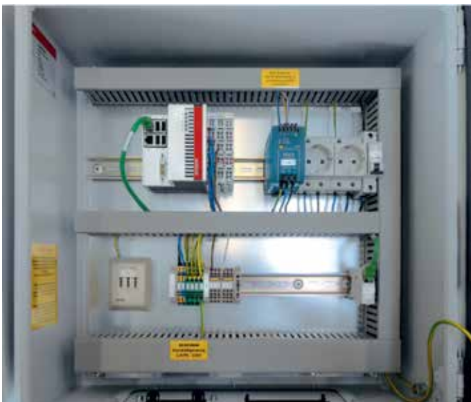
The data logger used in Aachen, Germany is approximately 40 cm in height and width, requires little space, and can be installed as an integrated solution with minimal effort. (Photo courtesy Beckhoff)
