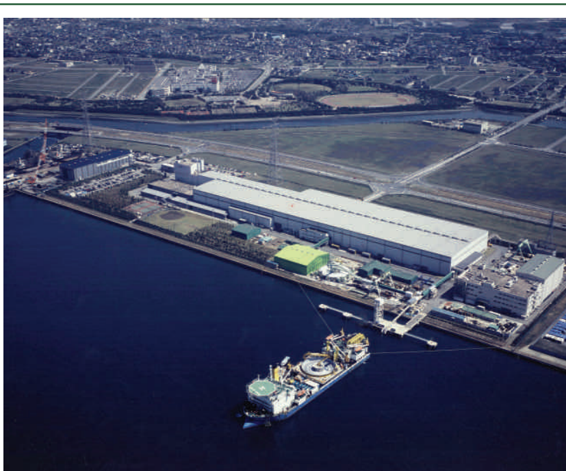
▲ The Nexans site in Japan where the cable will be manufactured
