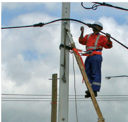
▼ Figure 10: Installation of aerial multi-duct assembly
