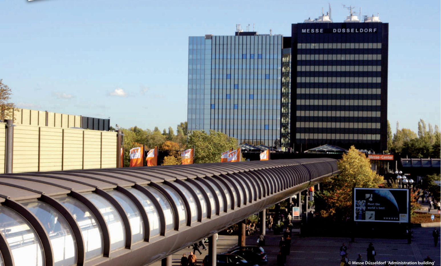
© Messe Düsseldorf 'Administration building'
