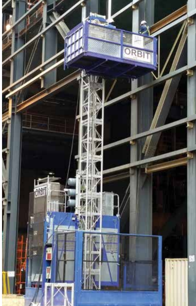
The Orbit personnel and material hoists' cages operate simultaneously.
