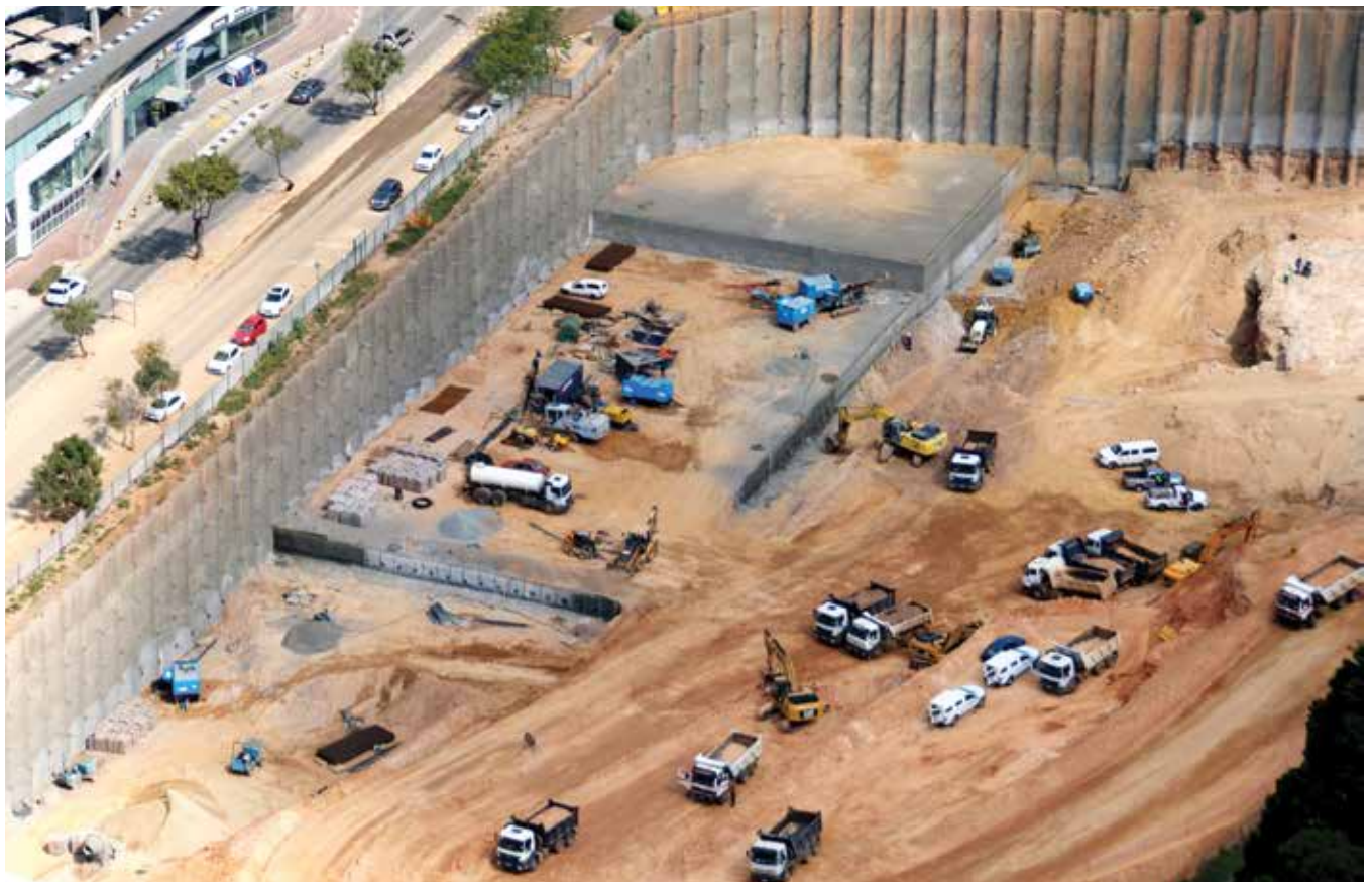
Completion of inner gunite walls over the Gautrain servitude.
