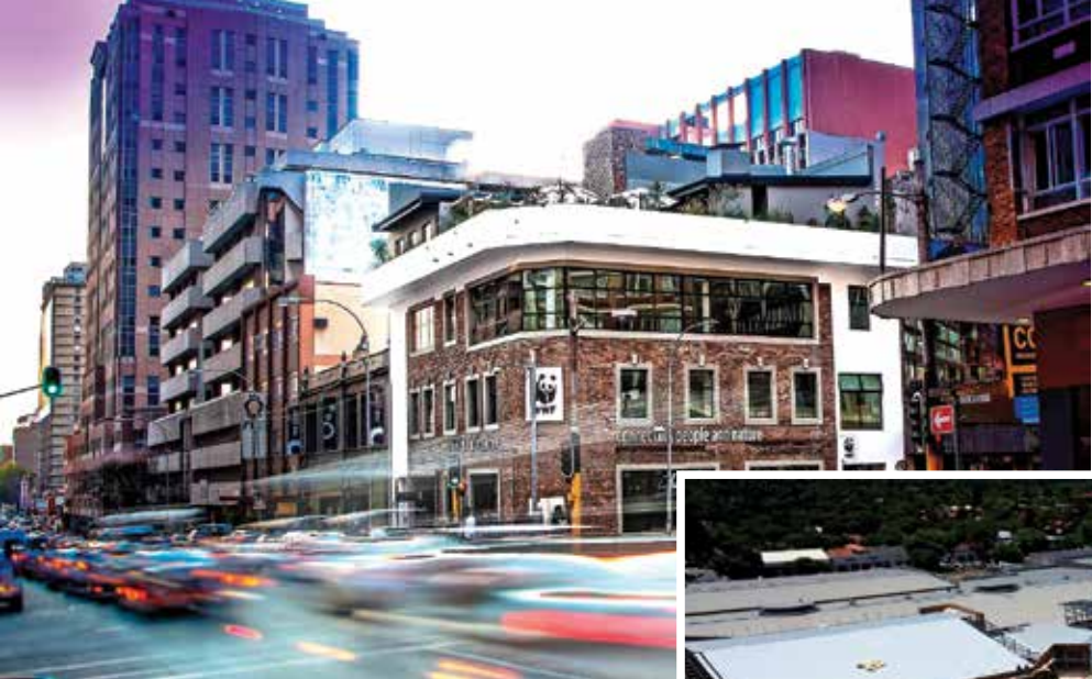
LEFT: The new WWF offices, in Johannesburg, is one of the group's latest office developments.
