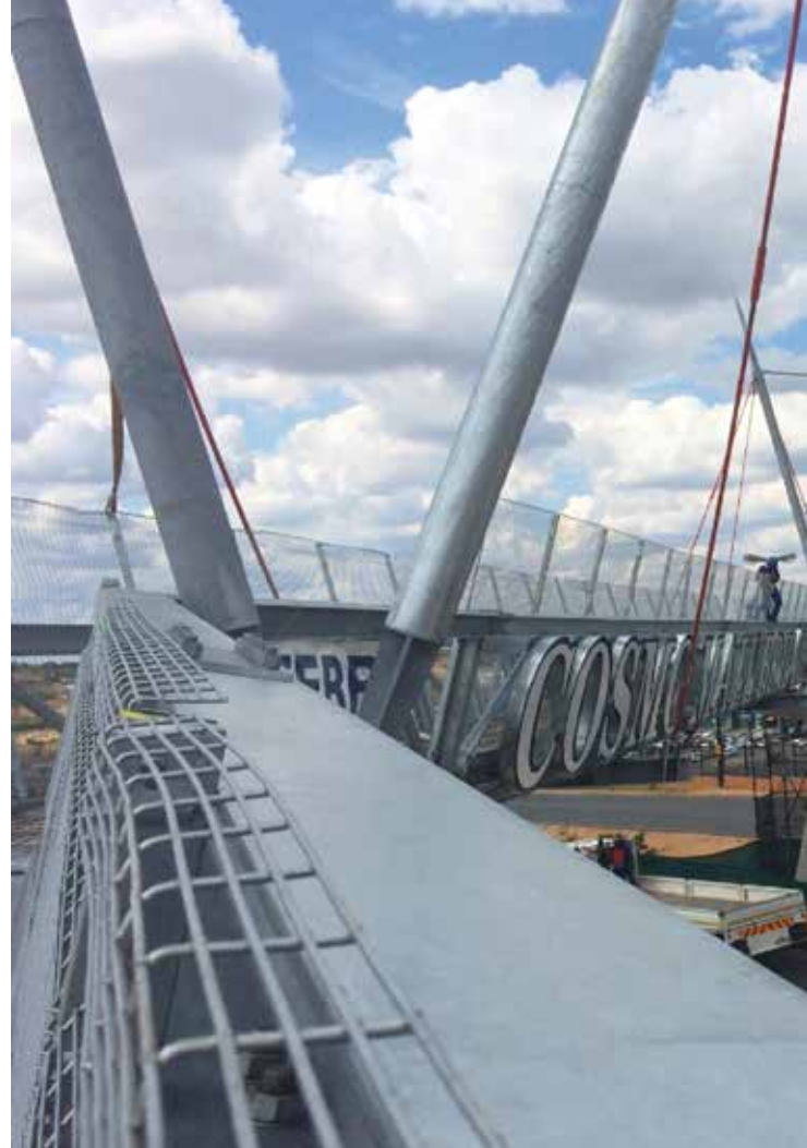
The Cosmo Pedestrian Bridge during construction.
