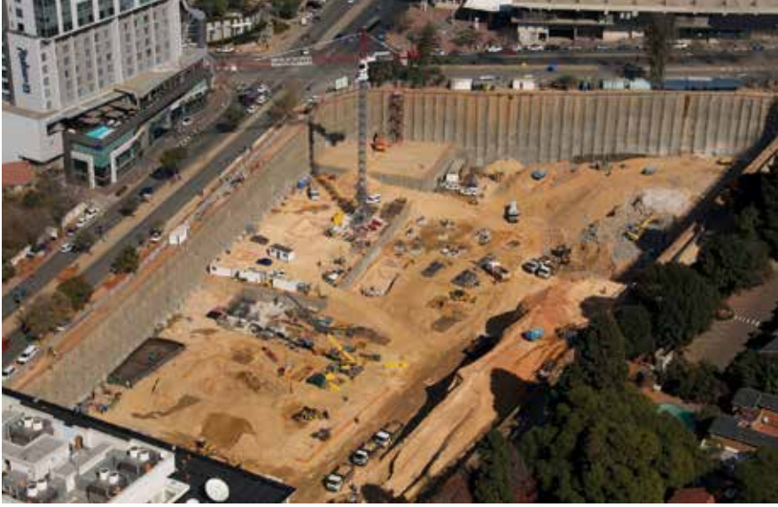
ABOVE: Phase I was handed over to the building contractor with the Rivonia Road face complete and rock profile exposed on the West Street face. BELOW: Stepped platforms over the Gautrain servitude.
