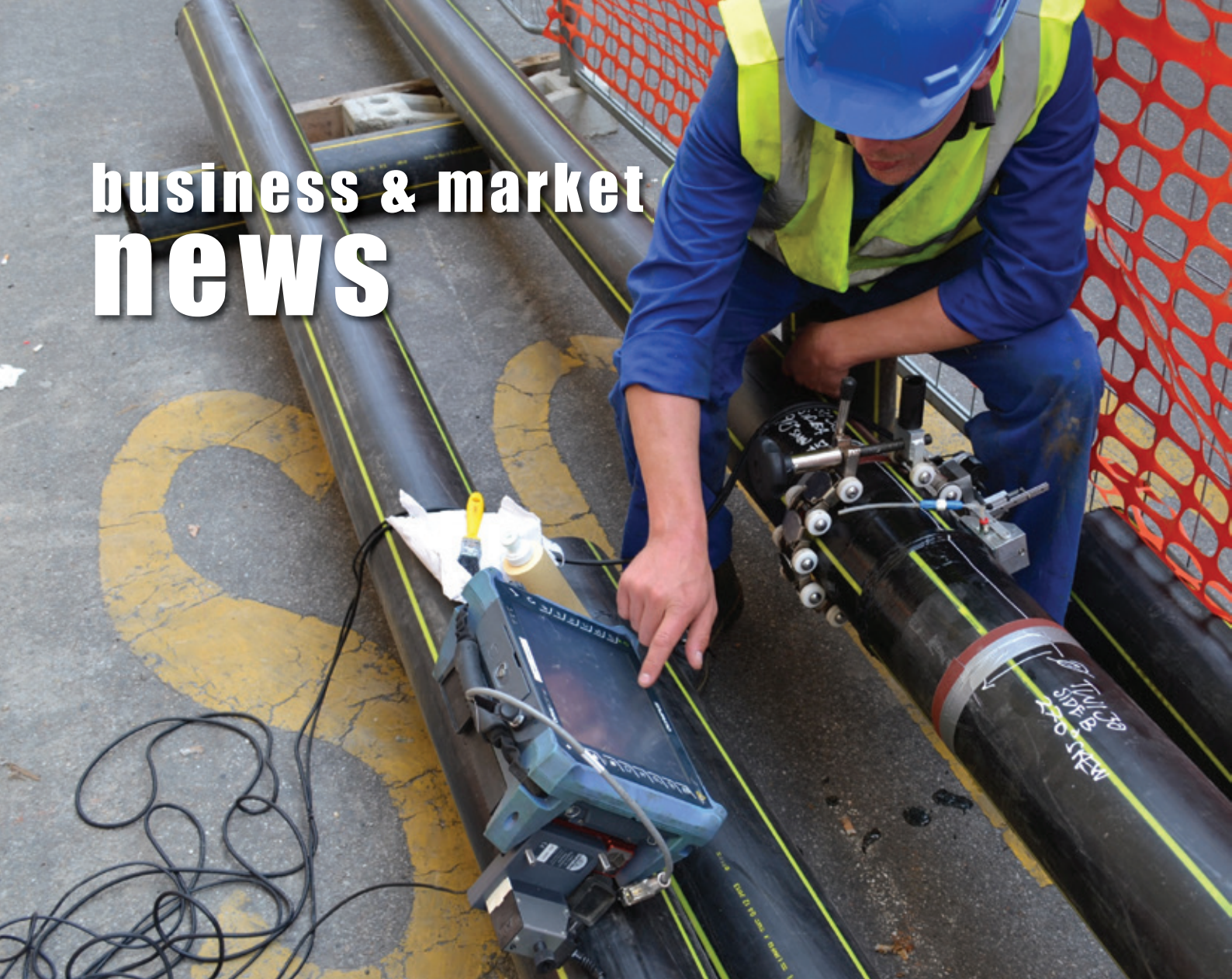
PolyTest system on-site inspection of a butt fusion joint in service
