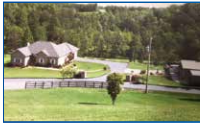
169 TWIN ROCKS LANE, LOWGAP - Custom built home by owner all on one level. Meticulously maintained. Hardwoods. Totally private two level deck with built in hot tub overlooking fenced pasture and stocked trout stream. Great view of Fisher Peak. Detached guest quarters/man cave. 16.76 acres! Private road shared with one neighbor..... $495,000
