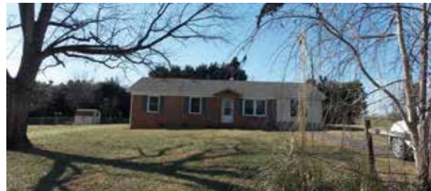
861809 - 108 Snow Hill Drive - Brick Ranch Style Home, Updated 3 BR, 2 Full Baths, Bonus Room that could be a 4th Bedroom, 2 Car Garage, New Appliances that Stay, New Roof, New Heat Pump & Air, Hardwood, New Carpet Floors, Patio, Corner Lot, Must See..... $118,500
