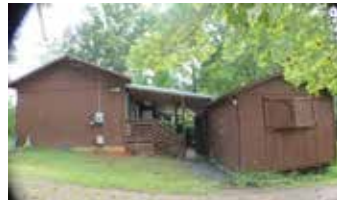
850932 - 202 ANNA BRYANT TRL - Wood floors and other materials were cut from the surrounding land. House has open kitchen, living area, dining area 1.5 BA, 2 BR and a detached screened in porch with storage on one end. HVAC system consist of individual Global Ductless Air Conditioner units in various locations throughout the house for a nice even heating and cooling. $67,900
