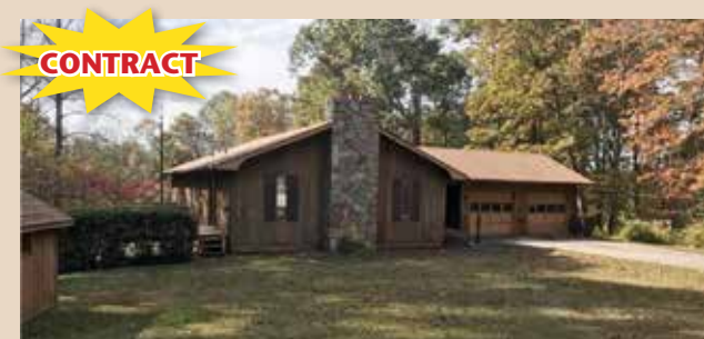
856906 271 TOMS CREEK RD., PILOT MTN. - Beautiful home is nestled in the country but is only 2 miles from Pilot Mtn. 2.11 acres w/ blueberry bushes, apple trees, a pear tree & a small greenhouse. 3 BR's, 2 full BA's w/double vanities & laundry on main. Lg. finished room in bsmt could be den, office or playroom. Lots of potential to finish the entire bsmt. Insulated windows, attached 2 car garage & deck..... $199,900
