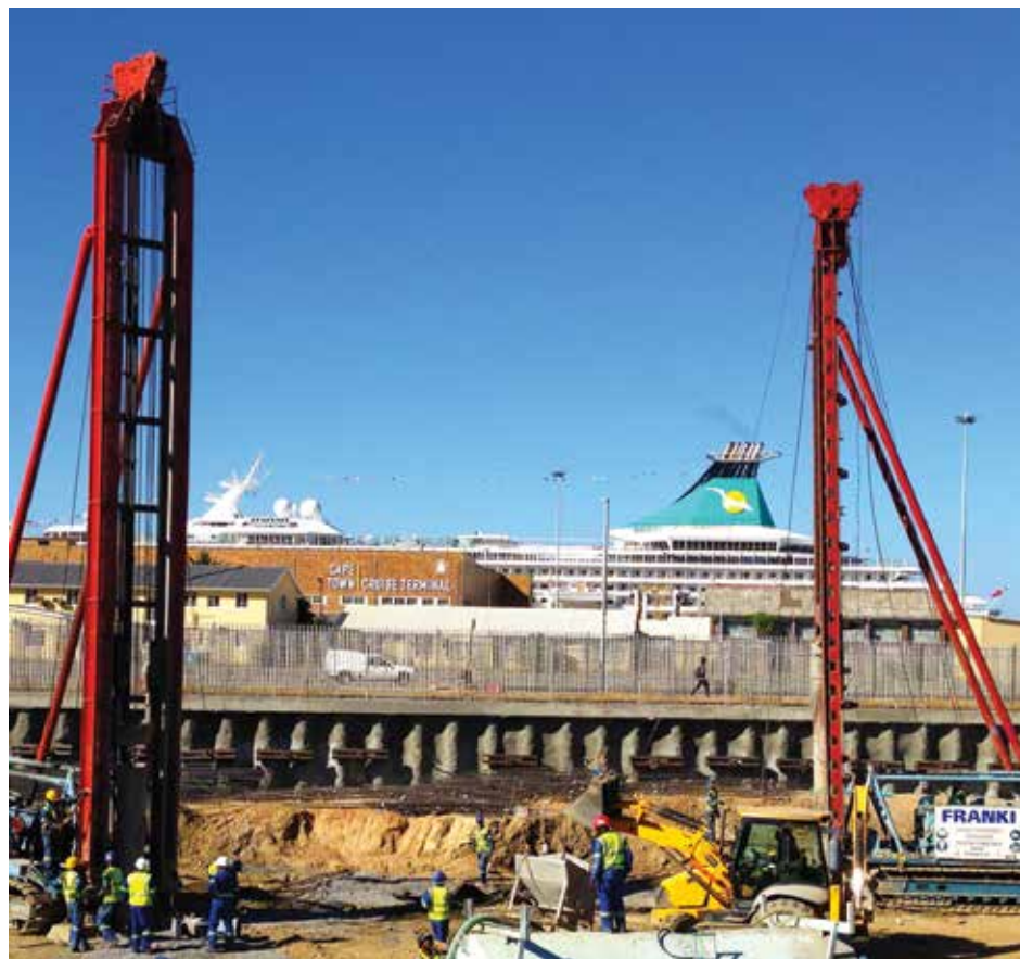
Installation of Franki Piles.
