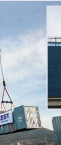
The super silent purpose built generator sets being lifted to the rooftop of the Christiaan Barnard Memorial Hospital.
