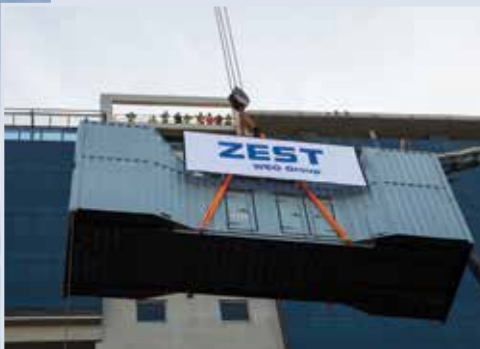
The super silent purpose built generator sets being lifted to the rooftop of the Christiaan Barnard Memorial Hospital.
