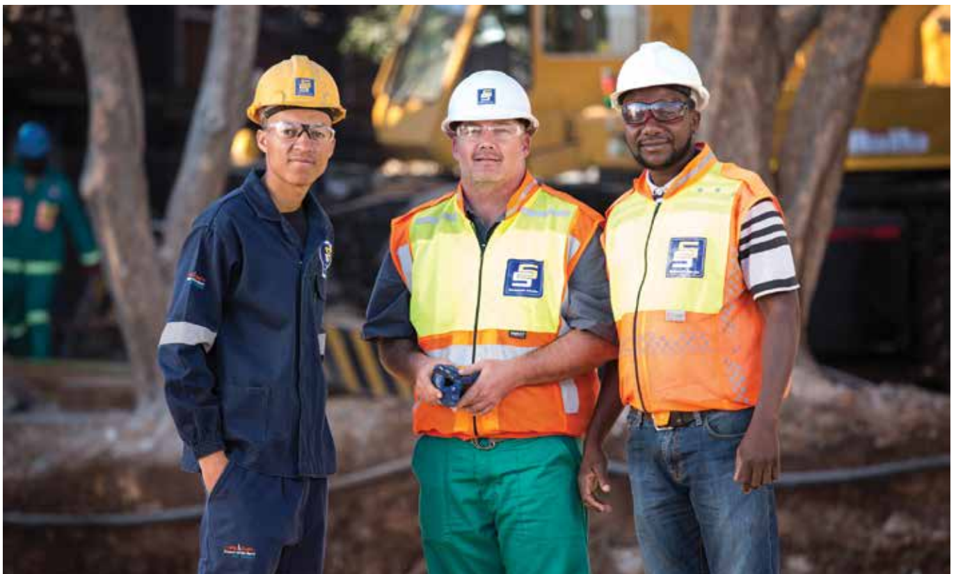
Pictured at a sinkhole rehabilitation project site in Centurion are, from left, Morgan Bentley, Johan Barnard (site foreman) and Lucas Mugondo (site safety manager).
