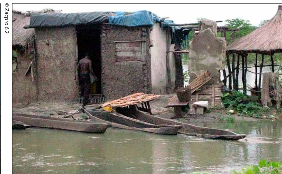
Destroyed homes following flooding in the Zambezi basin.
