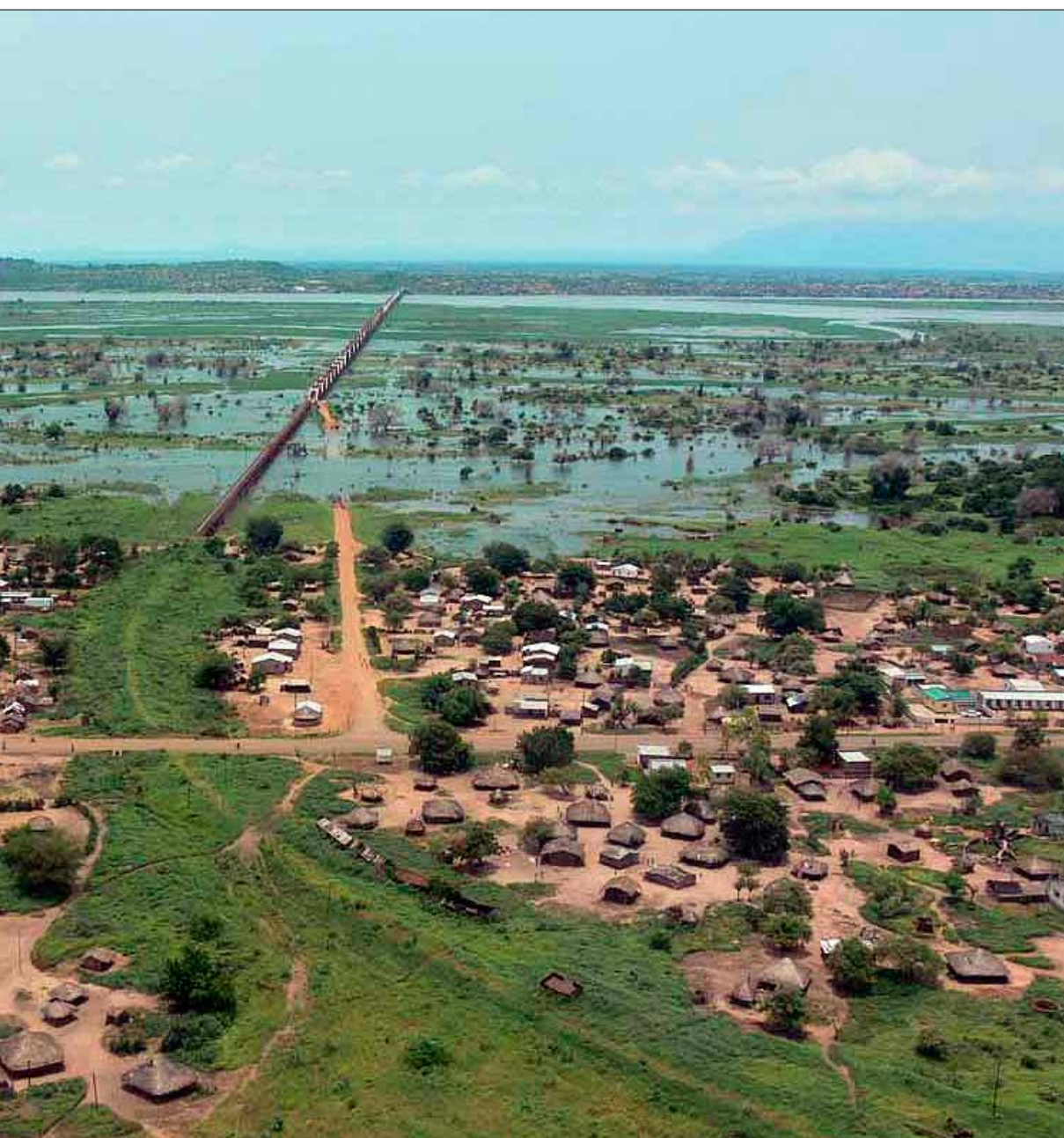
Sena- Mutarara flooding in Mozambique. Source: Ara Zambeze
