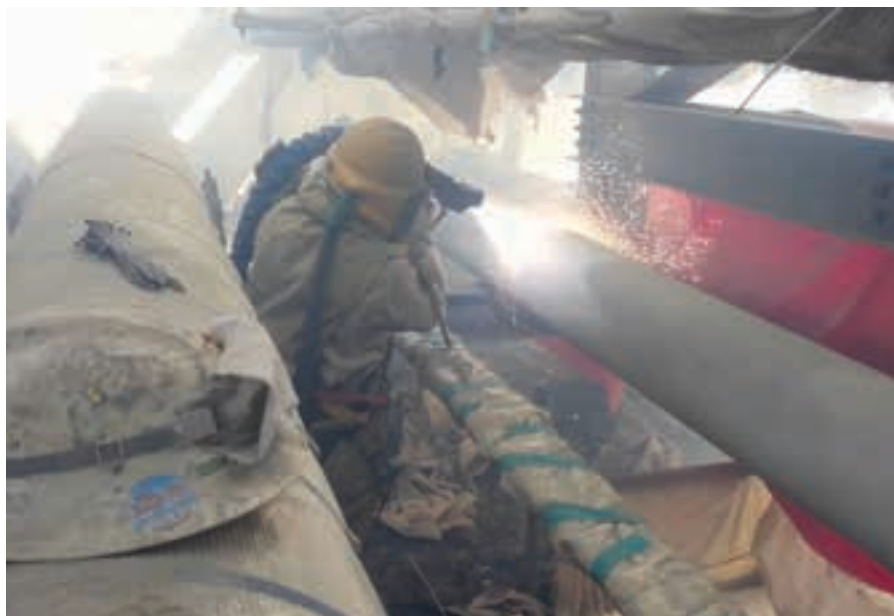
New and simple approaches to preventing CUI have recently emerged, such as the application of thermal spray coatings of aluminium onto the piping prior to insulating it.
