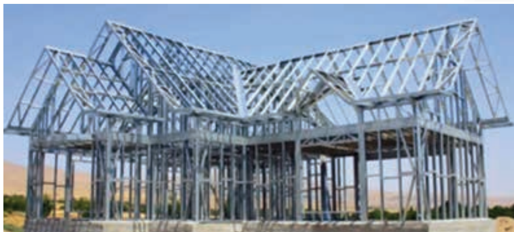
Light steel frame (LSF) building is a cost-effective construction method, with savings emanating mainly from time savings to completion, less rework, reduced logistical costs and a drastic reduction of rubble on sites.
