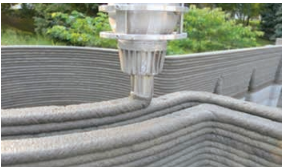
Construction is well suited to 3D printing as much of the information necessary to create a building will exist in CAD as a result of the design process.
