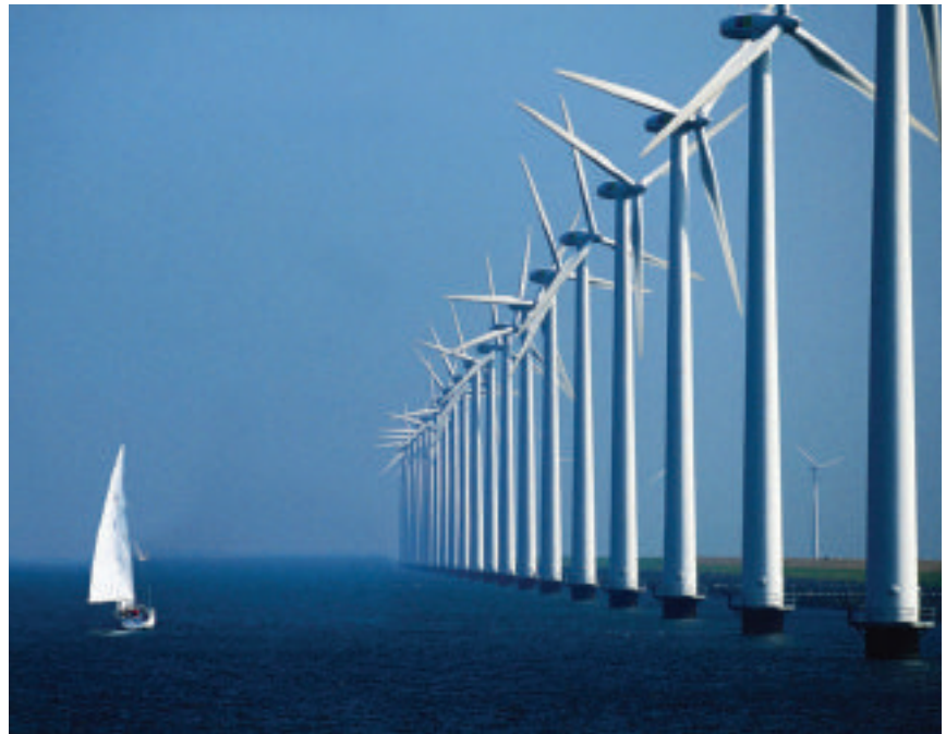
▲ An artist's impression of the completed Sheringham Shoal Offshore wind farm, off the Norfolk coast
