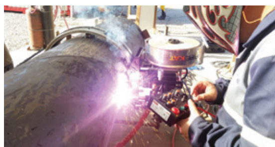
Pipe KAT in operation on a pipeline in Brazil
