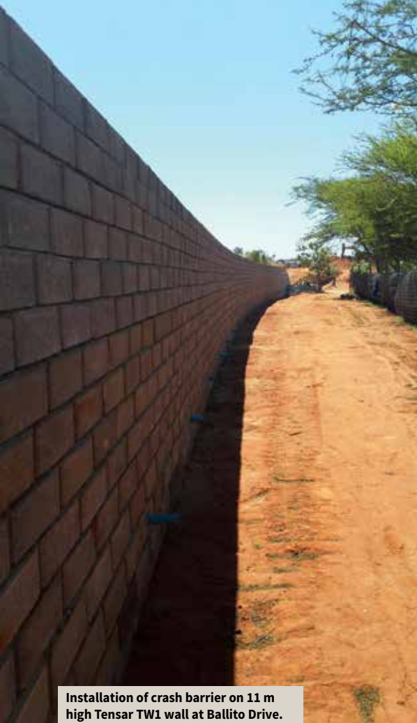
Locally manufactured Tensar TW1 blocks on 5 m high wall section.
