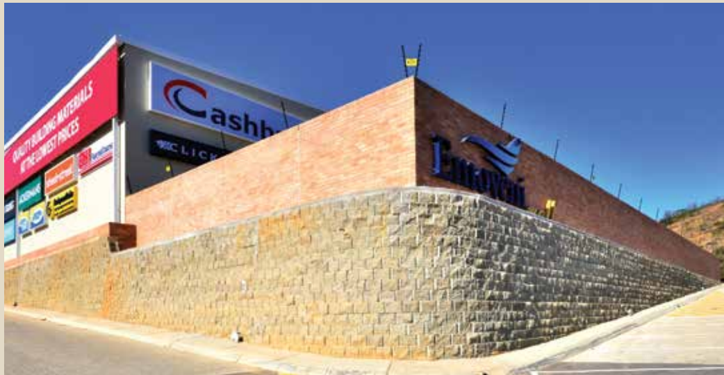
ABOVE AND TOP RIGHT: One of the closed-face walls built with Aveng Infracrete’s Infracrete™ 350.
