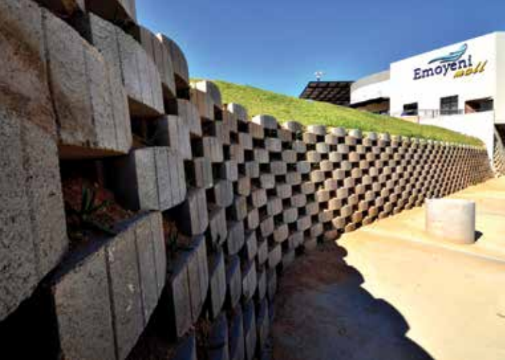
One of the open-face retaining walls at Emoyeni Mall.
