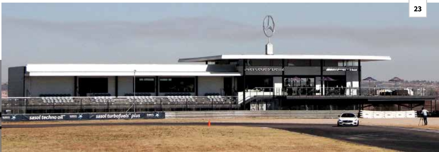
BELOW: The completed refurbished building pictured from the visitors' parking area, and also from the Zwartkops Race Track.
