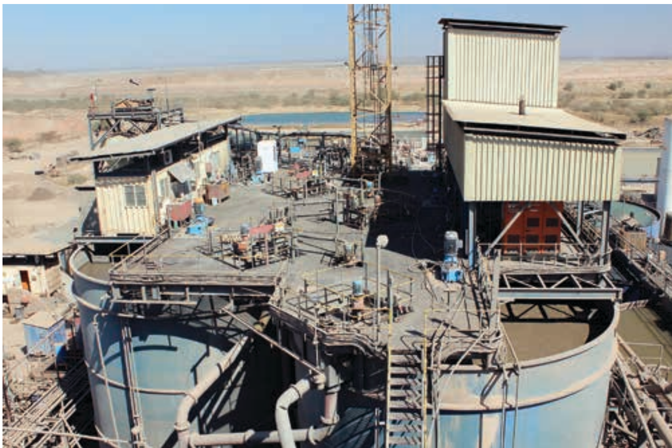
The Mupane processing plant, commissioned in 2004 and still going strong. It can process up to 1,2 Mt/a.
