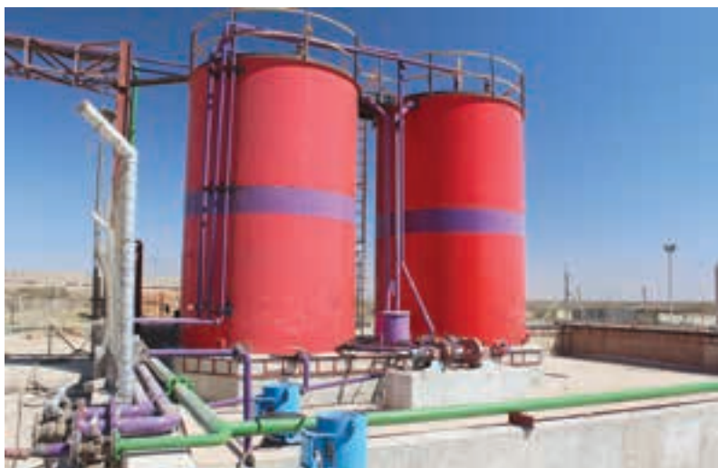
Recent enhancements to the Mupane plant include this liquid cyanide facility, expected to lead to a 1% increase in recovery.
