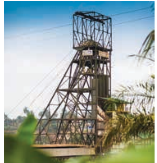
Headgear of the Prestea underground mine in Ghana, one of the oldest mines in the country. Golden Star is planning an open-pit operation on the Prestea property (photo: Golden Star).
