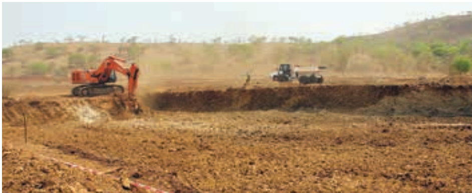
Earthworks in progress for the boxcut at Yaramoko (photo: Roxgold).
