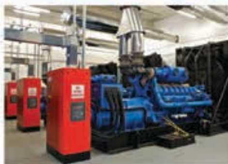
Six 2 000 kVA open type synchronising generator sets
