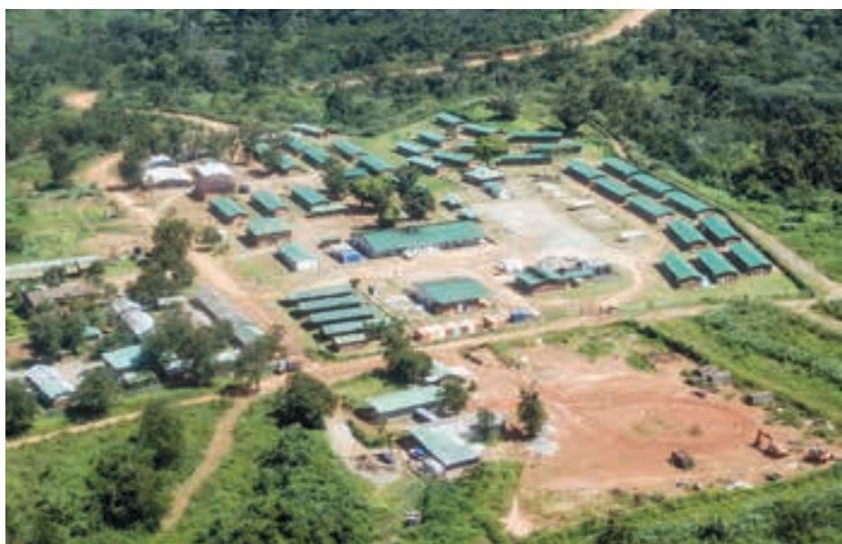
The Namoya mine camp with employee housing, canteen and some offices.
