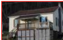
MLS# 58855 ~ Fries, VA ~ 2 Bed 1 Bath Overlooks New River ~ Most Updating Done but Needs Some Interior Finishing Work & Roof ~ Great Price! ~ $49,900
