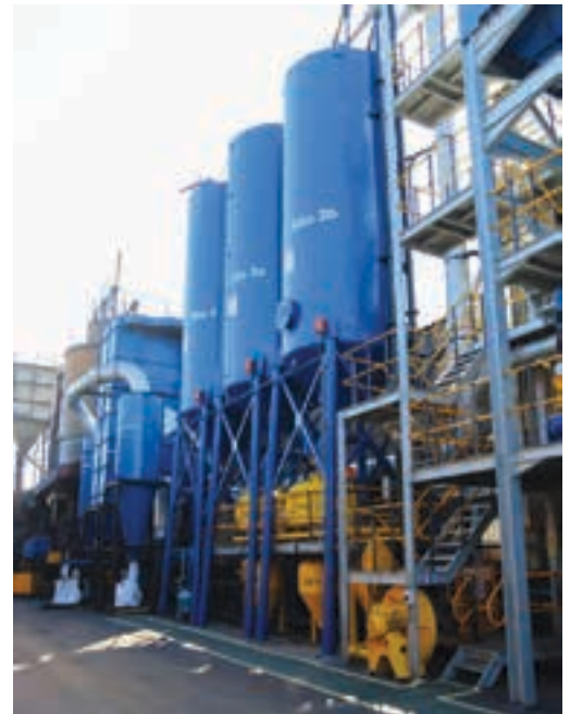
The newly installed sand plant at Weir HBF.
