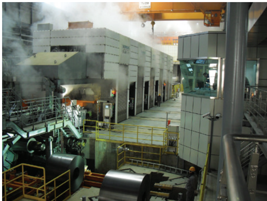
Cold rolling mill from Primetals Technologies at Tangshan Iron and Steel Group
