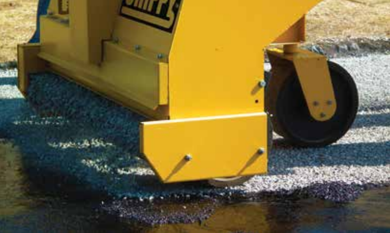
The company's hand operated chip spreader, known as Chippy, has been acknowledged by the Construction Industry Development Board as a very effective method of undertaking single and double seals using labour-based methods.
