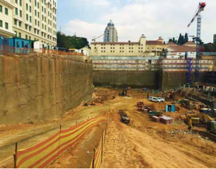
Lateral support being concluded on the western face below the Balalaika Hotel.
