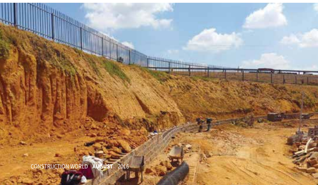
The lower wall under construction at The Grove.
