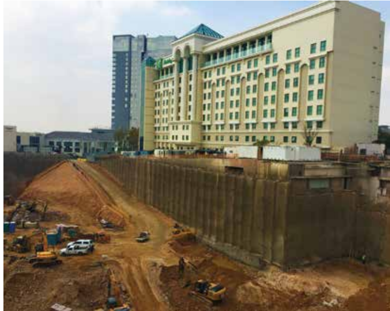
LEFT: Anchor drilling along Maude Street face, below the contaminated material area. RIGHT: Lateral support walls in close proximity to the Holiday Inn Hotel.
