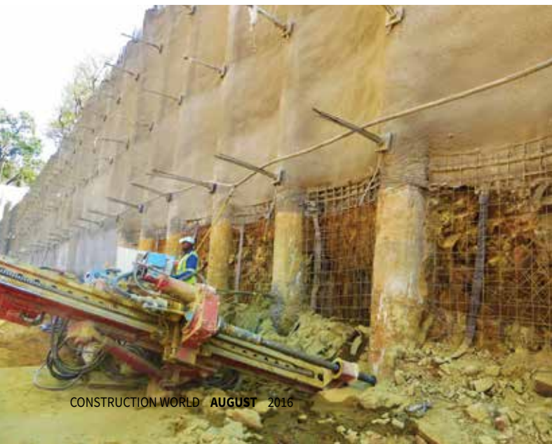
LEFT: Anchor drilling along Maude Street face, below the contaminated material area. RIGHT: Lateral support walls in close proximity to the Holiday Inn Hotel.
