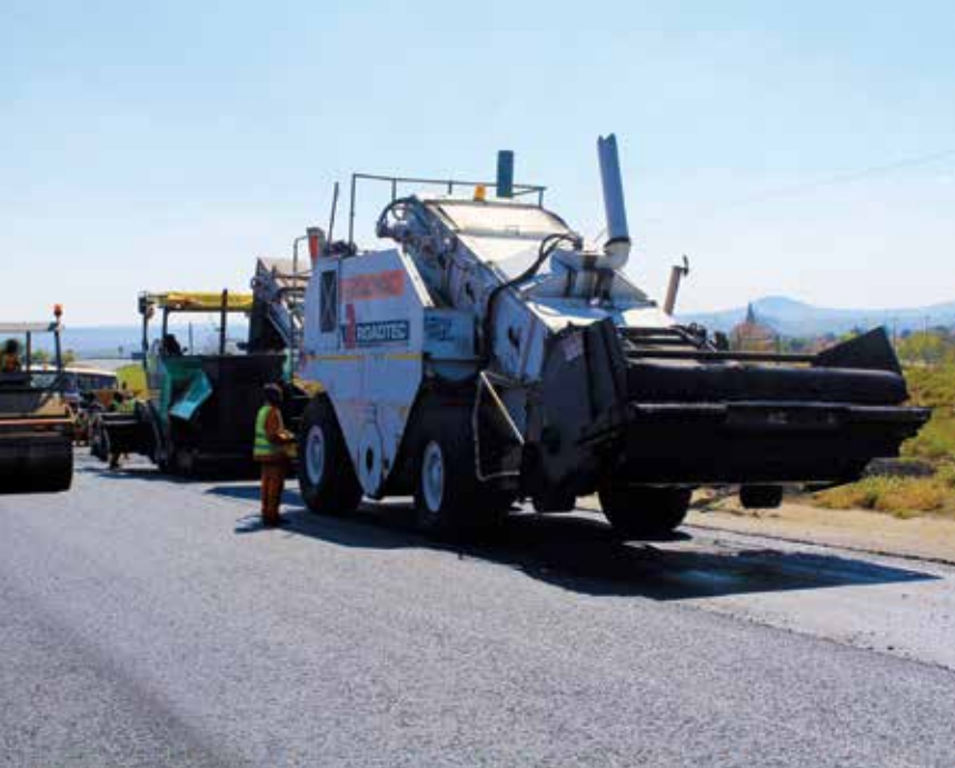
Roadmac Surfacing has deployed three paving teams on this project.
