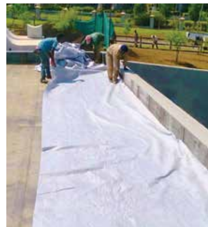
The final bidim A2 layer separates the cover soil from the woven tape underneath.
