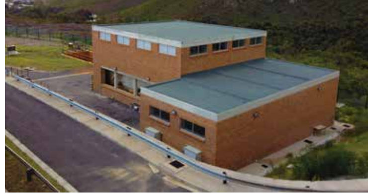
2015's winner in the Professional Services category for Best Projects was Aurecon for its work at the Preekstoel Water Treatment Works.
