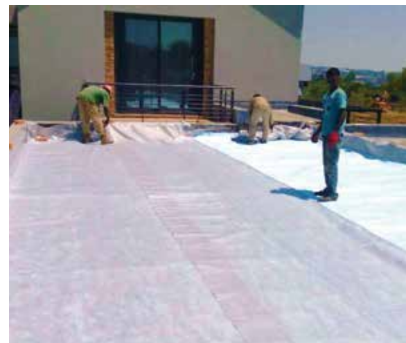
The final bidim A2 layer separates the cover soil from the woven tape underneath.
