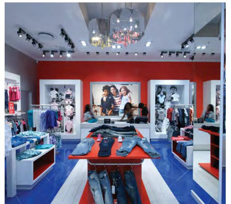
An energy efficient LED solution that fits the brand aesthetically, looks modern, is low in maintenance, and reduces the in-store heat load while complementing the strict international lighting and store design levels required by the retail brand.
