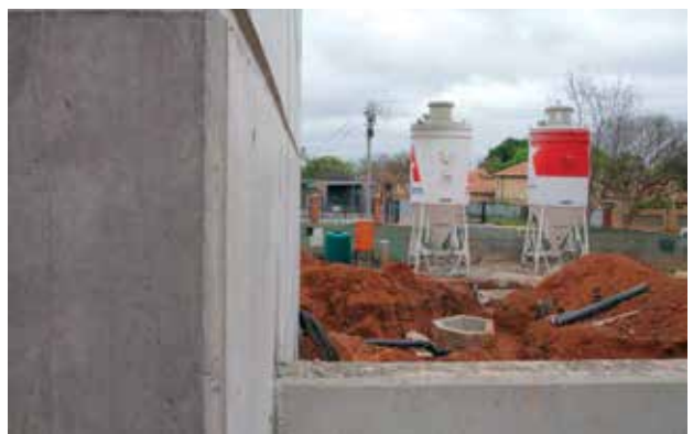
The Class II mortar has been specially engineered as a dual purpose mix that can be used for both mortar and plaster work. BELOW: AfriSam's Dry Mortar product can be delivered in 10 or 20 ton silos to meet customer and project requirements.
