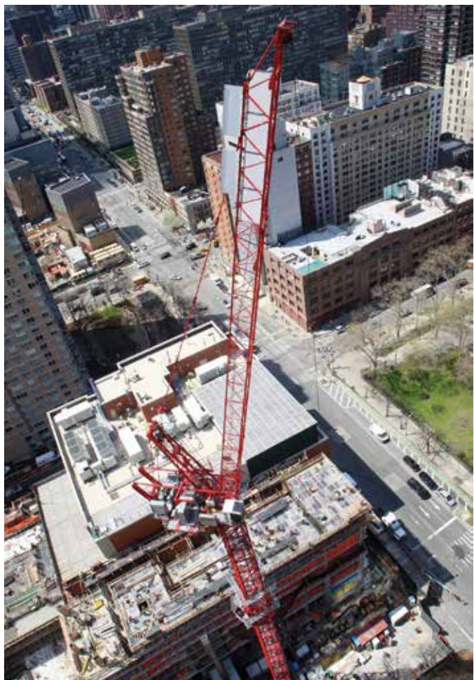
BELOW: The Potain MR 418 is the first in an updated line of luffing jib cranes, each of which is equipped with full frequency-controlled mechanisms for precision control.
