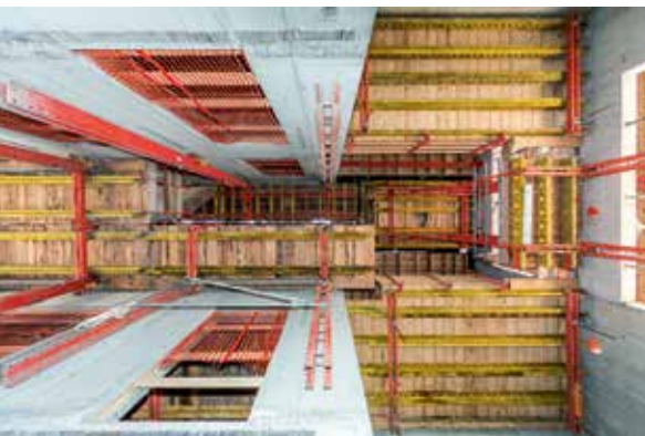
The PERI climbing formwork solution for the high-rise core was based largely on the crane-independent working RCS Rail Climbing System, combined with a self-climbing ACS Platform Unit as well as crane-climbed CB Climbing Platforms and BR Shaft Platforms. BELOW: In addition to ensuring short striking times, the SKYDECK Panel Slab Formwork also allowed easy adaptation to match the slab geometry which changed from storey to storey.
