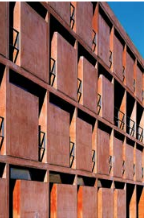
The use of pigmented or coloured concrete showcases it as an aesthetically pleasing and modern building material.
