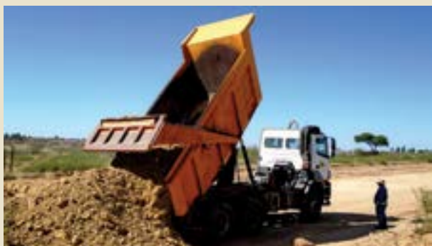
A tipper truck tipping fill material onto the road area.
