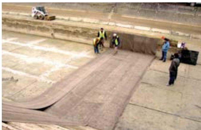
It can be used to rapidly reline and refurbish existing concrete structures suffering from environmental degradation and cracking.
