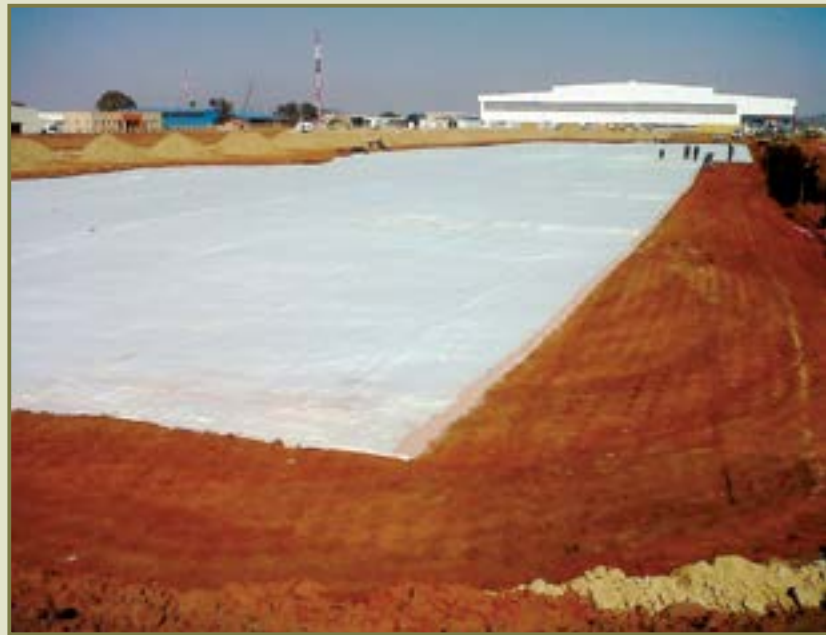
The 29 000 m 2 of Rockgrid PC was used to reinforce the substrate.
