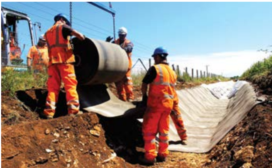
Concrete Canvas can be rapidly unrolled to form a channel lining.
