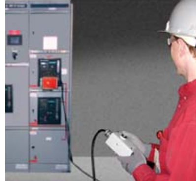
Remote Racking Device
