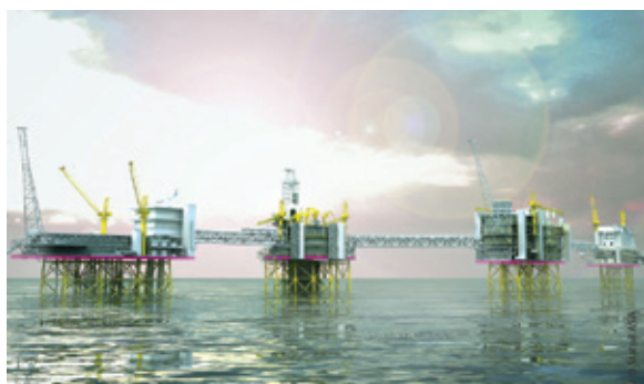
The first phase includes erecting four platforms
