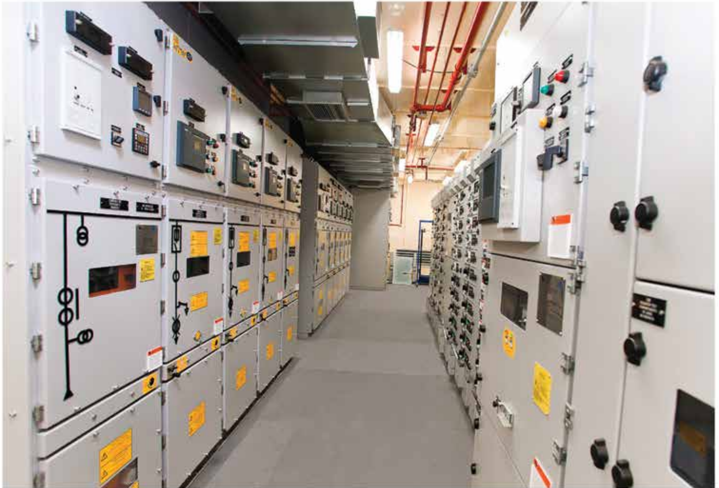
LV and MV Switchboards inside "E" House
