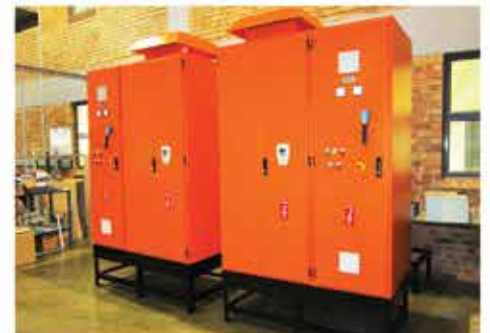
CFW Family Variable Speed Drive
