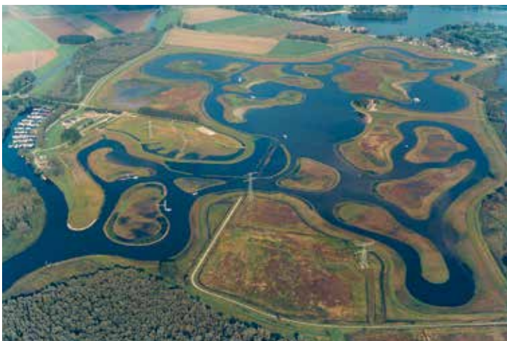
left SEVILLE, SPAIN Maintenance dredging and removal of the top layer of the construction pit for the future lock in the commercial river port of Seville.
