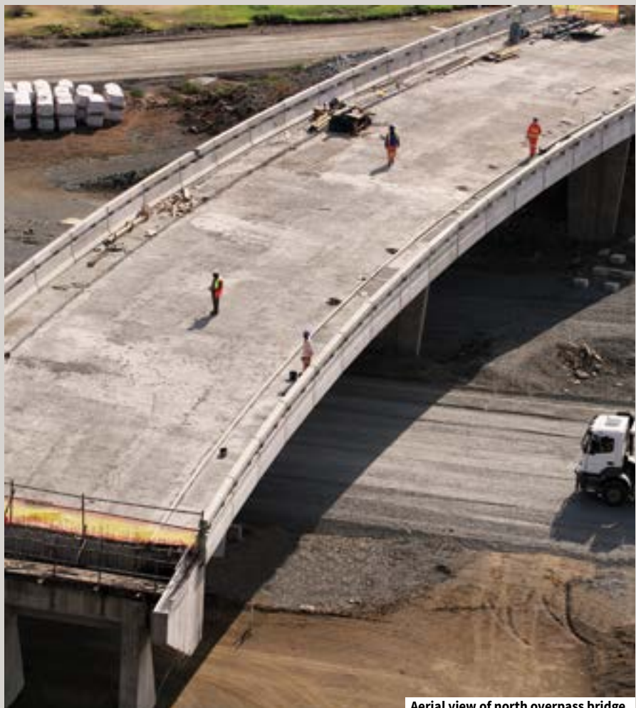
Aerial view of north overpass bridge.
