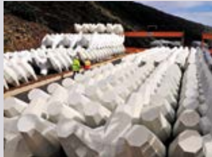
LEFT: About 700 litres of Chryso's products have been shipped 2 300 km across the South Atlantic Ocean to St Helena. RIGHT: Over 700 units of precast Core-loc armour units (7 tonnes per unit) and hollow blocks (27 tonnes per unit before filled with stone) were placed by crawler cranes via GPS around the wharf from the surface bed to just above sea level.
