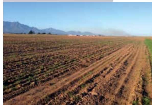
RESA 11 (Runway End Safety Area) upon practical completion of the project.
