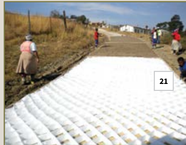
Local labour was used to fill the Multi-Cell road
