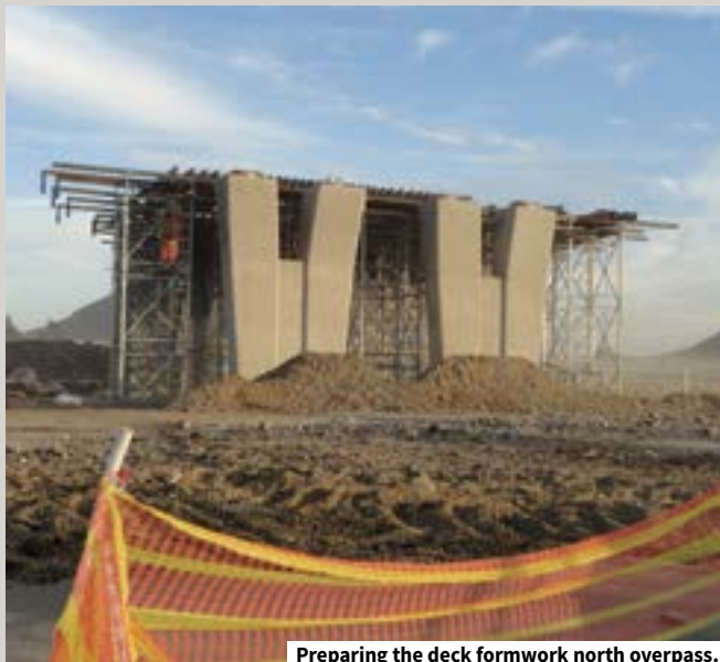
Preparing the deck formwork north overpass.
