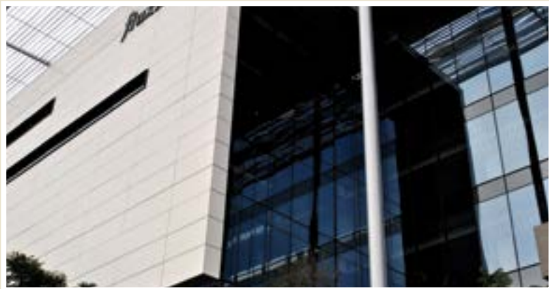
Dow Corning’s new 896 Panel Fix system was used for the façade cladding of the new 30 Jellicoe Avenue office block in Rosebank. a.b.e.-approved applicators, Rudolph & Van Vuuren, factory-produced the composite ceramic panels, bonding them into aluminium frames before transport to site for final installation.
