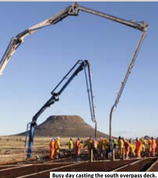
Busy day casting the south overpass deck.
