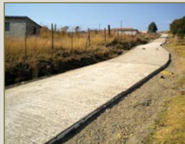
The completed road ready for foot traffic and small vehicles.
