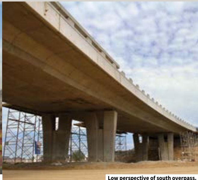
Low perspective of south overpass.
