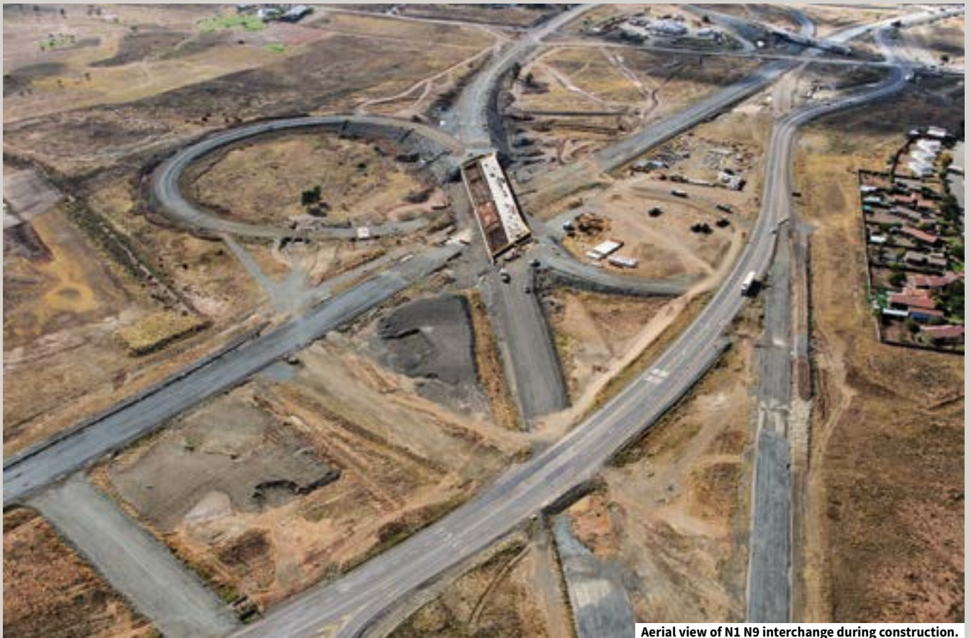
Aerial view of N1/N9 interchange during construction.
