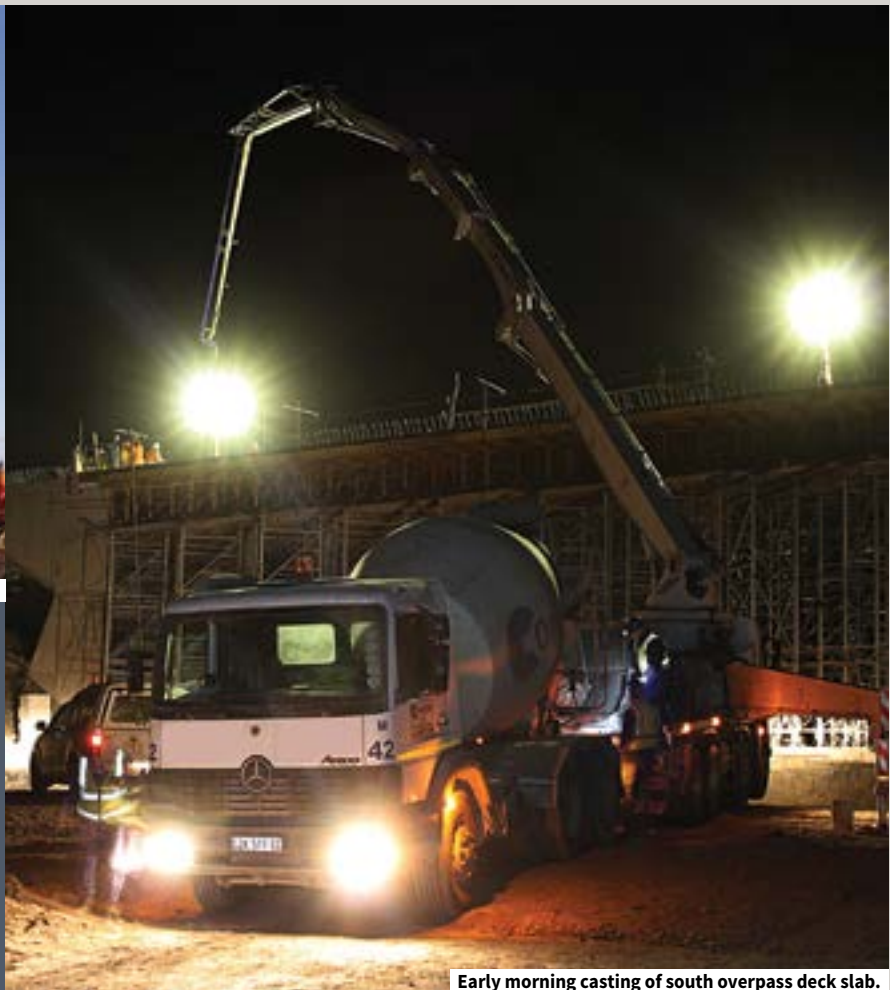
Early morning casting of south overpass deck slab.
