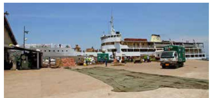
Ferry loading terminal, Mwanza, Tanzania
