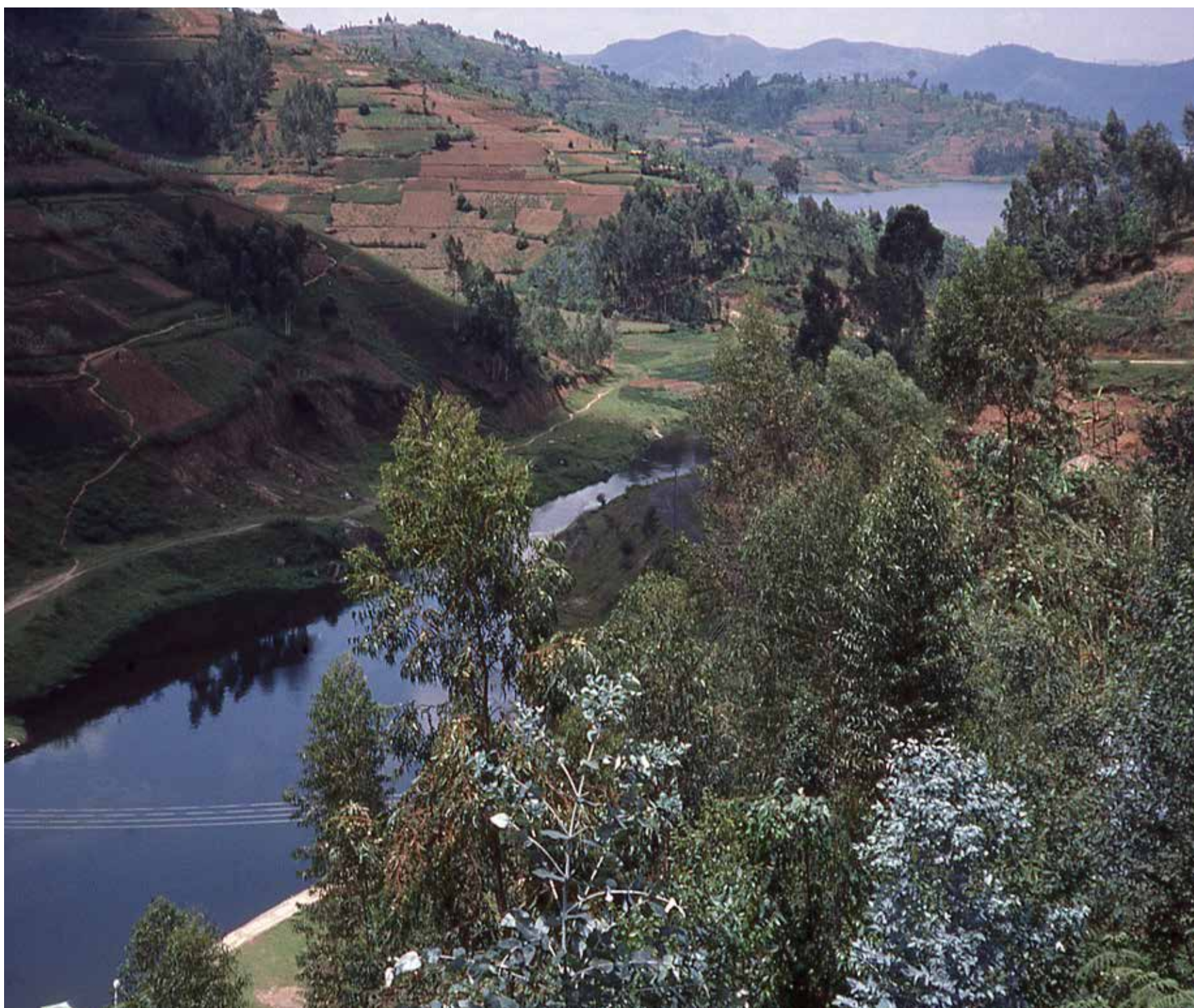
Hydro generation plant between Lake Ruhondo and Lake Burera, Rwanda
