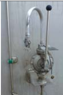
Dewater/sampling pump installed with anti-siphon valve for operation from ground level
