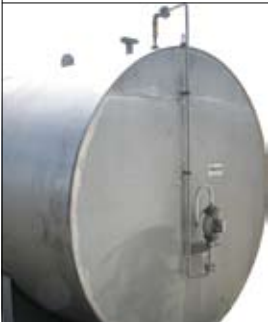
Dewater/sampling pump installed with anti-siphon valve for operation from ground level
