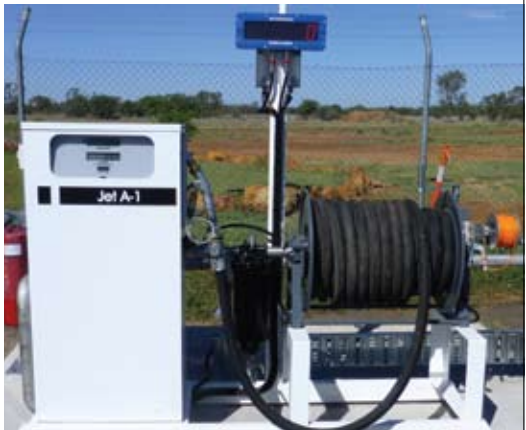
Dispenser system with overwing and single point refuelling, high visibility register.
