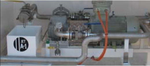
Self-bunded storage tank with on-demand pump system and emergency backup refuelling equipment
