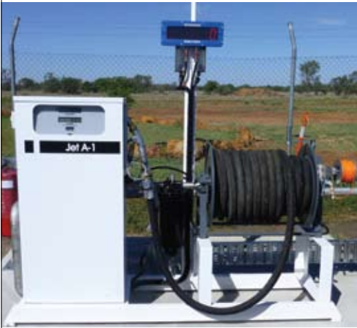
Dispenser with high capacity hose reel, filter, static reel and over and under wing refuelling nozzles.
