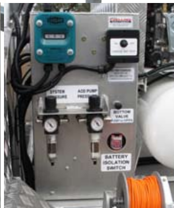
Pneumatic controls and tank overfill protection system.
