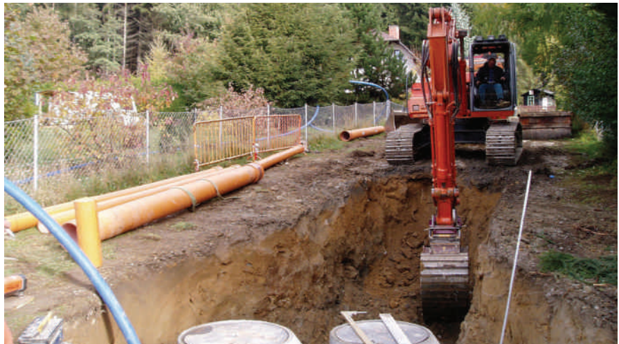
i The low weight of pipes made from BorECO PP allows fast and cost-efficient pipe laying
