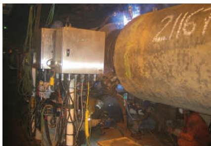
Eight TransPuls Synergic 3200 pipe welding systems simultaneously produce two cover layers on one pipe joint
