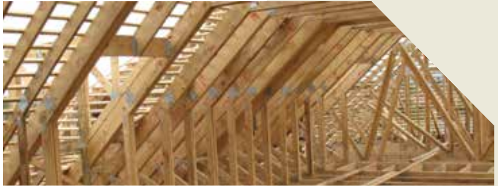
Prefabricated timber roof trusses
