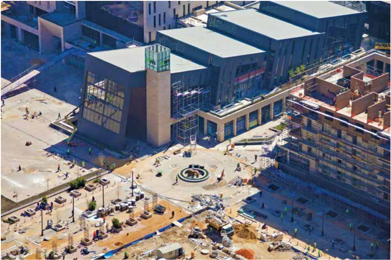
An aerial view of Menlyn Maine during construction.
