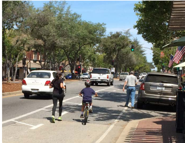
Figure 2-4: Monterey Road narrowed to one lane in each direction. The second lane is repurposed as a buffered bicycle lane
