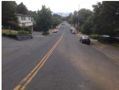
Figure 1-19: Del Monte Avenue
