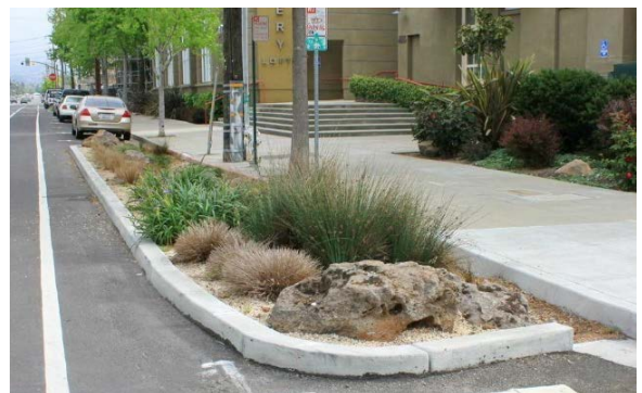
Figure 2-19: Example of planted bulb-out between parking spaces
