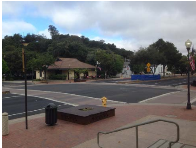
Figure 1-33: Crosswalk with brick pavers and in-pavement flashers installed at unsignalized intersections
