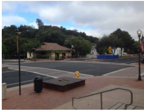
Figure 2-6: Crosswalk with brick pavers and in-pavement flashers installed at unsignalized intersections
