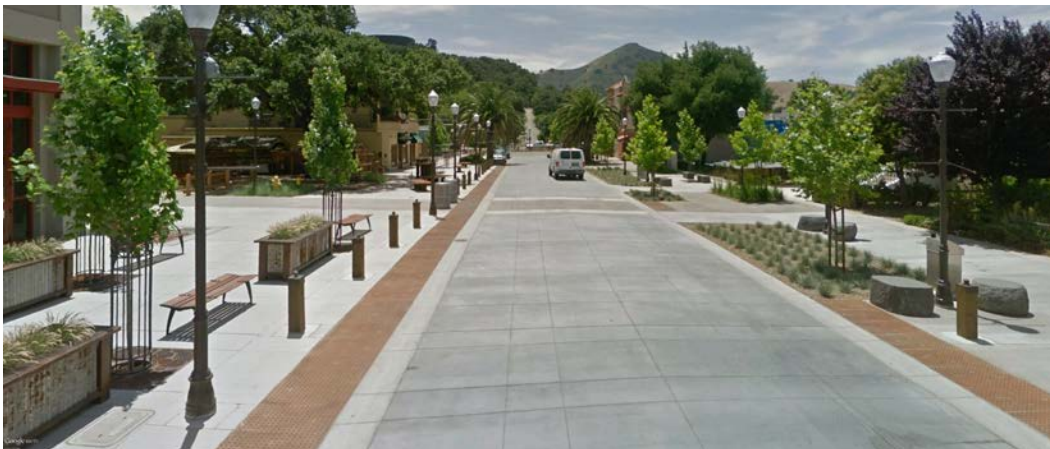
Figure 1-22: Shared Street between Morgan Hill Transit Center and Downtown. Source: Google Streetview
