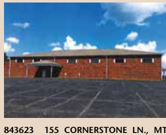
843623 155 CORNERSTONE LN., MT. AIRY - 12,600 s.f. brick & block building w/ shingle roof, covered entrance basketball gym w/kitchen, restrooms w/shower, dining hall, mezzanine w/storage & mechanical room. Built in 2000. An additional 7,700 s.f. metal bldg. currently used as a worship center. Covered entrance to lobby w/tile floor, drop ceilings, restrooms, offices, break room, meeting rooms & more. Propane gas heat. Built in 1989..... $950,000
