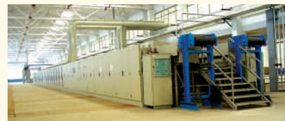
○ High safety requirements from CPA
