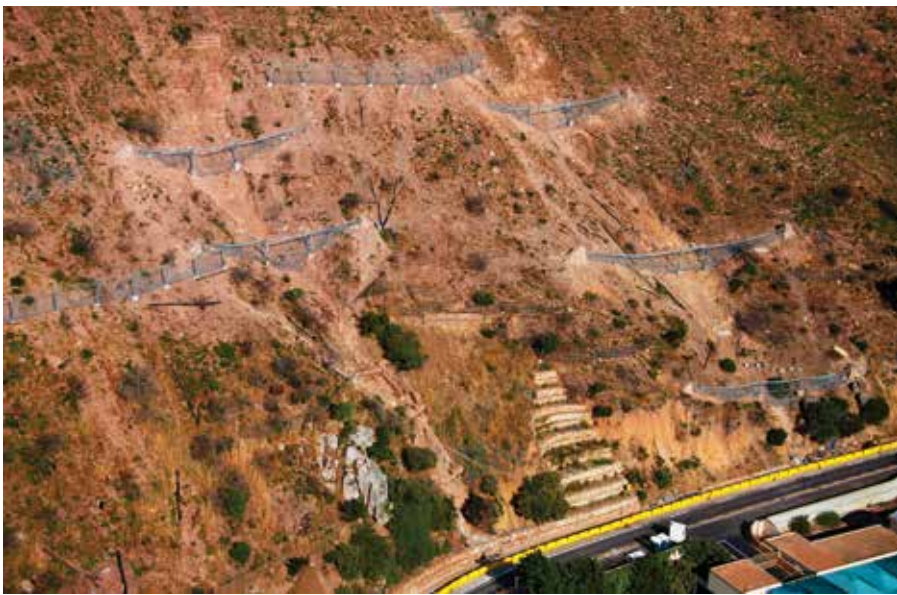
Aerial view of the completed fences.
