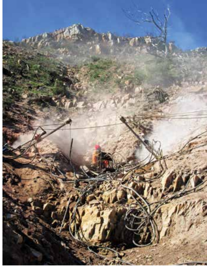
Difficult drilling in the northern gully for debris flow fence.
