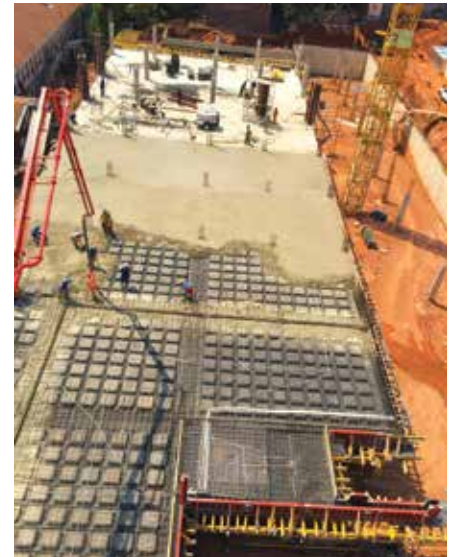
LEFT: Concrete bleed and plastic shrinkage crack. RIGHT: CHRYSO® Macro Fibres (pictured) provide effective post crack control in concrete once it has hardened while CHRYSO® Micro Fibres provide effective crack control in concrete during the pre-hardening phase. BELOW: CHRYSO® Macro Fibres were used in all of the surface beds for the basement and parking areas of the new consulting rooms for the Zuid-Afrikaans Hospital in Pretoria.
