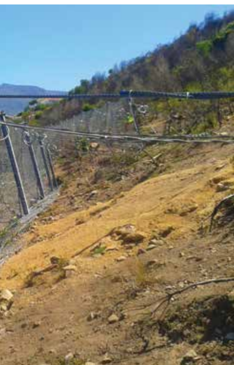
BELOW: Landslide fence.
