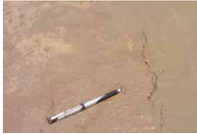
LEFT: Concrete bleed and plastic shrinkage crack. RIGHT: CHRYSO® Macro Fibres (pictured) provide effective post crack control in concrete once it has hardened while CHRYSO® Micro Fibres provide effective crack control in concrete during the pre-hardening phase. BELOW: CHRYSO® Macro Fibres were used in all of the surface beds for the basement and parking areas of the new consulting rooms for the Zuid-Afrikaans Hospital in Pretoria.
