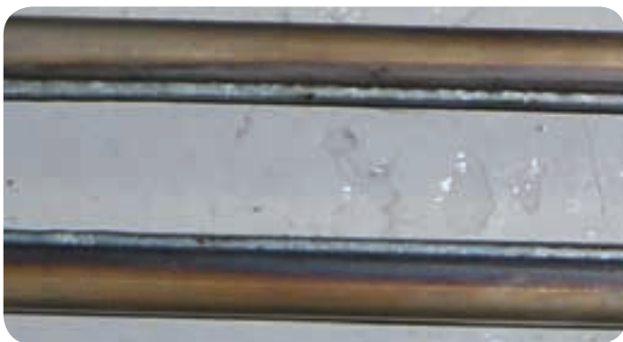
Figure 16: A comparison of the visible HAZ on typical LSND (top) and conventional MAG welded (bottom) beam parts manufactured in the trial.
