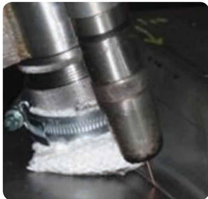
Figure 10: The LSND welding system, with coolant seal in place, in situ on a top-hat weld joint shown trailing the robotic MAG welding torch.
