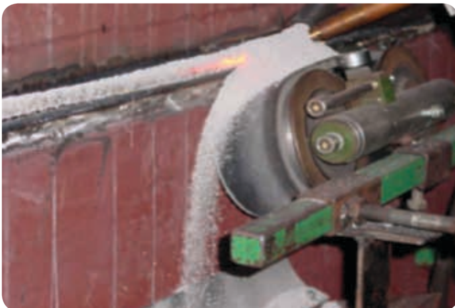
Horizontal-vertical submerged arc welding of a tank.
