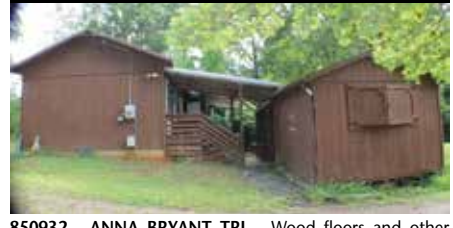
850932 - ANNA BRYANT TRL - Wood floors and other materials were cut from the surrounding land. House has open kitchen, living area, dining area 1.5 BA, 2 BR and a detached screened in porch with storage on one end. HVAC system consist of individual Global Ductless Air Conditioner units in various locations throughout the house for a nice even heating and cooling. $82,100
