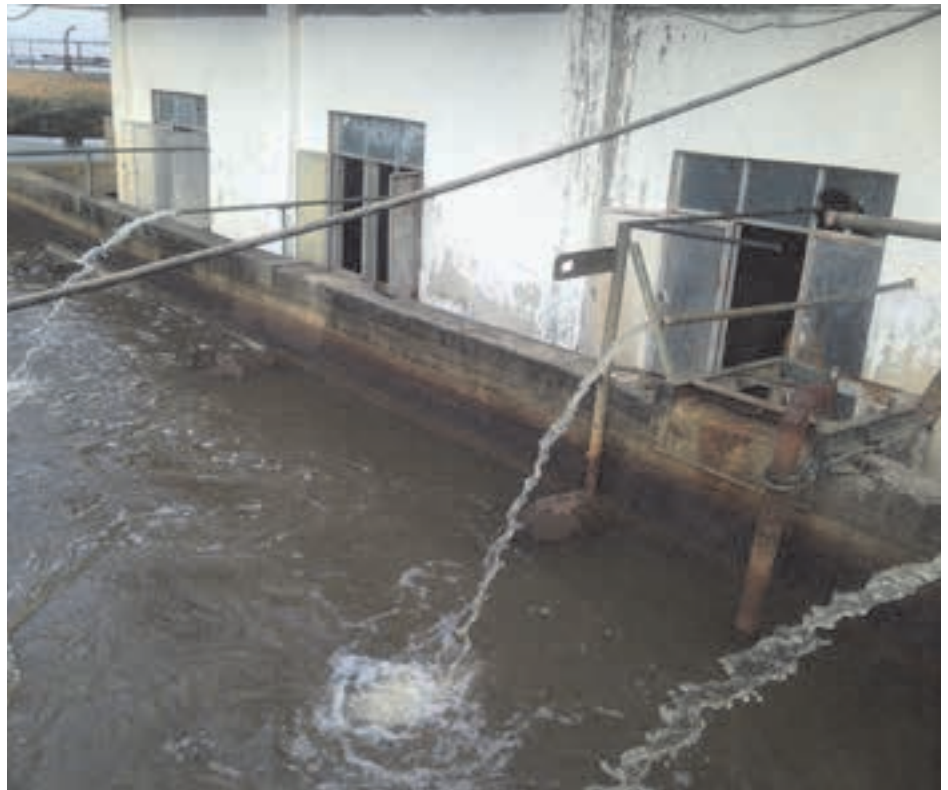
Figure 2: Plant operators found that if they left the vent pipes open during normal pumping operation, the stream of water back into the hot well was a visible means of identifying any loss of priming.
