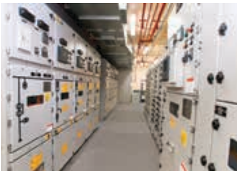
LV and MV Switchboards inside E-House
