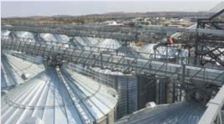
SAB’s first fully automated and connected maltings plant will produce 150 000 tons of malt every year.
